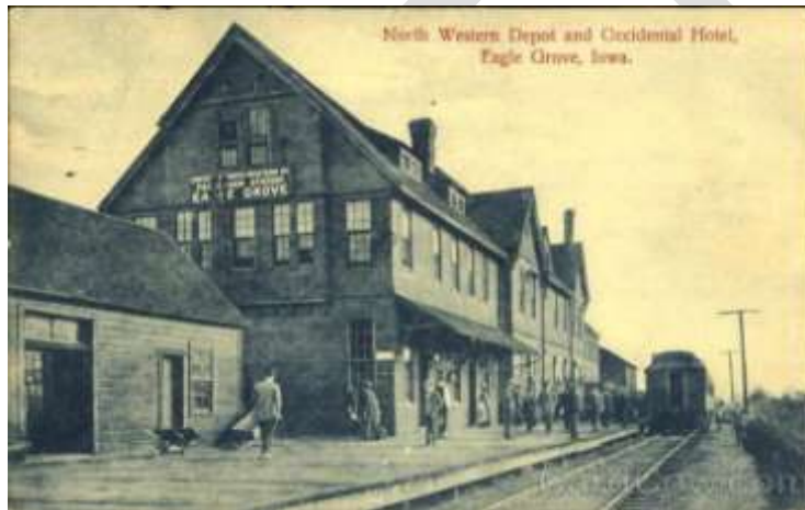
Figure 2.3: Northwestern Depot - Eagle Grove, IA
