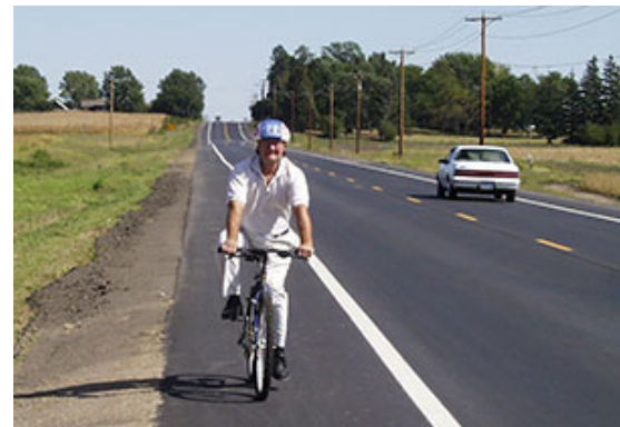
Paved Shoulder along a State road
