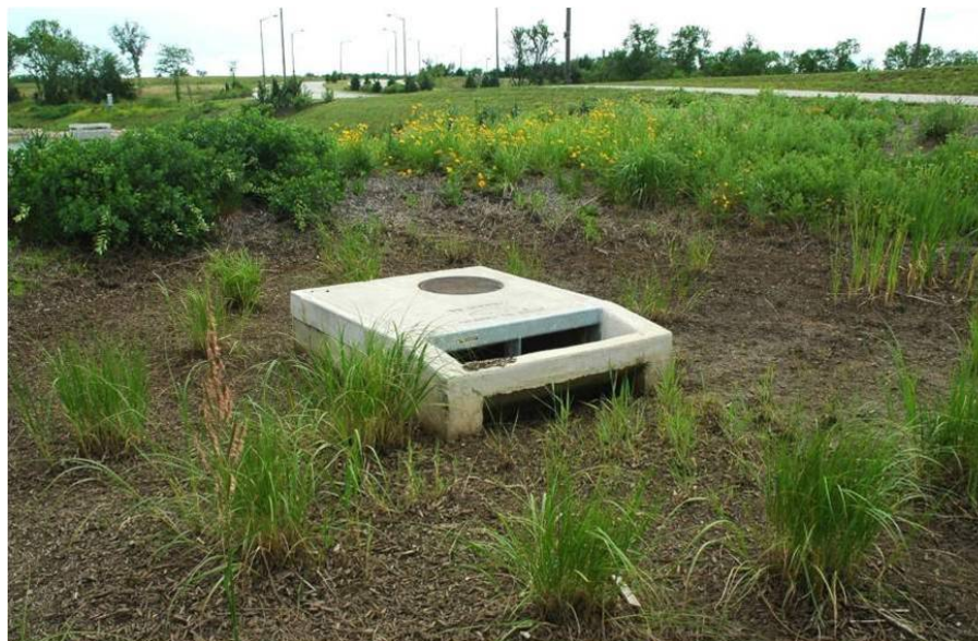
Figure 4-12 Mize Lake, Lenexa, Kansas Bioretention High Flow Structure
