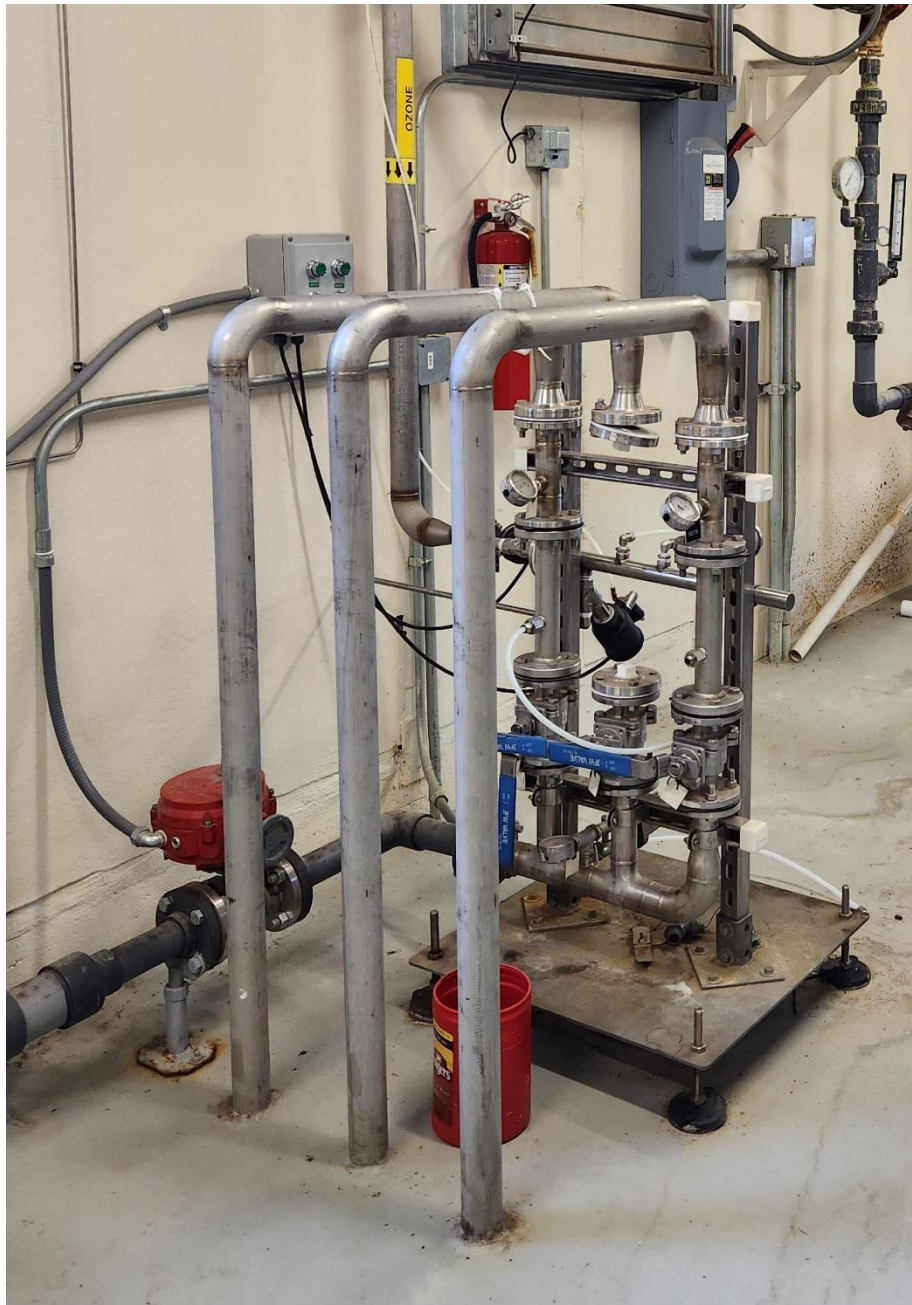
Figure 7: Ozone Ejector Skids
