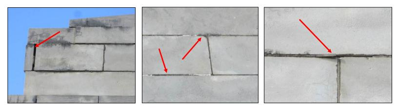
(4) The vertical head joints between all coping stones shall be cut back a minimum of ½-inch in depth, cleaned of all loose and foreign debris and then resealed utilizing a polyurethane rubber sealant, Masterseal NP100 or equal. Bond breaker tape shall be installed into the bottom of the cut joint to prevent three-sided adhesion. New sealant shall be tooled to a neat, uniform appearance and shall match the existing material in color as closely as possible.
