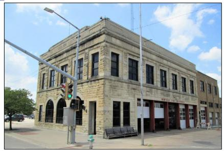
(1) All stone surfaces of the South and East elevations shall be washed with pressurized water at approximately 1000 PSI. Where necessary to remove stubborn stains, a chemical cleaning agent shall be applied to the surface, allowed to dwell, and then rinsed in accordance with the manufacturer's specifications. The chemical cleaning agents shall be applied no more than two times to any masonry surface.
