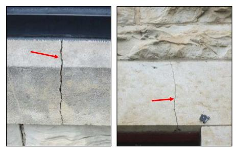
(7) The vertical joints between stone window sills, stone band and stone water table joints shall be cut back a minimum of ½-inch in depth, cleaned of all loose and foreign debris and then resealed utilizing a polyurethane rubber sealant, Masterseal NP100 or equal. Bond breaker tape shall be installed into the bottom of the cut joint to prevent three-sided adhesion. New sealant shall be tooled to a neat, uniform appearance and shall match the existing material in color as closely as possible.
