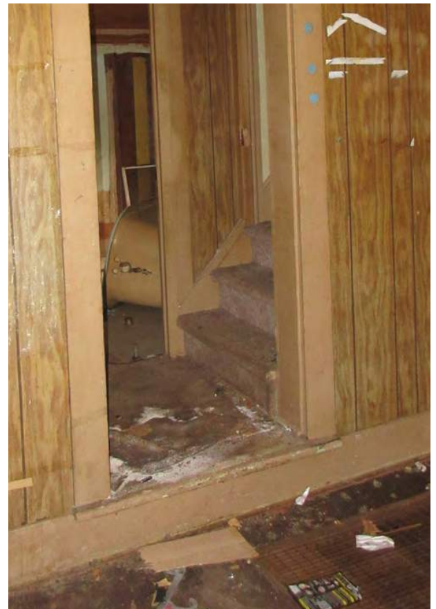
Figure 17: The image on the left depicts the carpet that is missing from the lower-middle steps in the stair case. The image on the right displays the white residue that has developed and a portion of the carpet that is missing at the base of the staircase.
