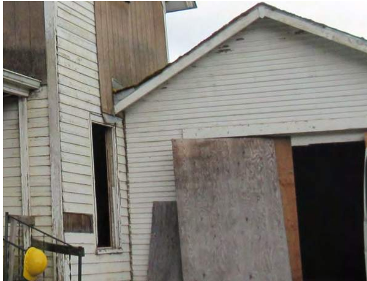
Figure 10: The first image above (left) exhibits the location where the cornerboard is missing at the juncture where the eastern façade of the garage meets the northern façade of the two-story structure. It also displays the paint chipping below the eave on the garage's eastern façade. The second image (right) depicts a close-up view of the vertical unpainted strip at the juncture along this eastern façade that suggests that a cornerboard had once existed there.
