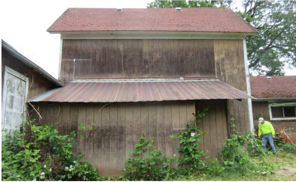
Figure 7: The image above exhibits a good example of the T-111 siding on the western façade of the main two-story volume and its attached shed that has accumulated water residue and lost a significant amount of color.
