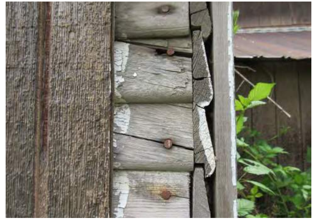
Figure 9: The image on the left displays the cornerboard that has been removed from the southeastern corner of the garage, and the image on the right displays the shiplap siding on this corner that shows paint erosion due to continuous water exposure over the past seven years.
