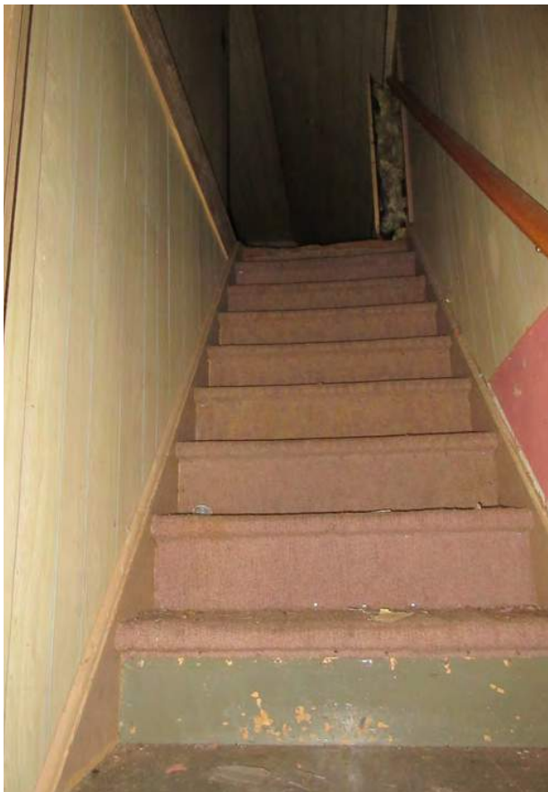
Figure 17: The image on the left depicts the carpet that is missing from the lower-middle steps in the stair case. The image on the right displays the white residue that has developed and a portion of the carpet that is missing at the base of the staircase.
