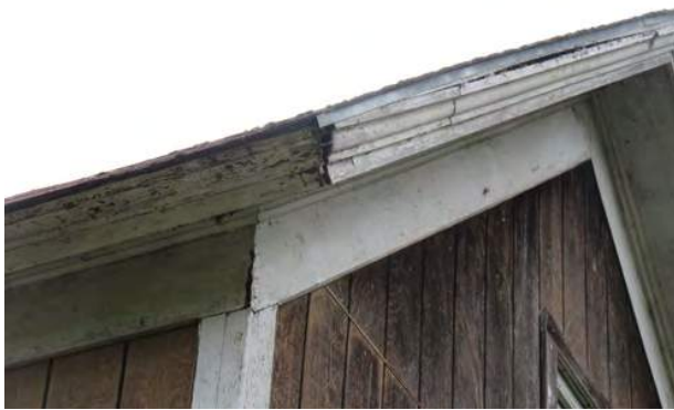
Figure 4 (left): The image above displays the tip of the cornice that is missing on the southern side of the two-story volume as well as the separation between the cornice and flashing on this edge. Figure 5 (right): This image depicts the loosely attached flashing on the southern roofline of the garage.
