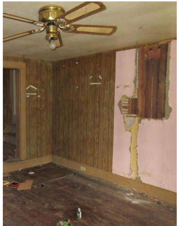
Figure 14: These images depict the living room in its current condition. Most pink wallpaper has been removed to reveal the underlying finishes, most notably around the fireplace. The final image depicts the damaged portion of the northern wall through which the dining room is visible on the other side.
