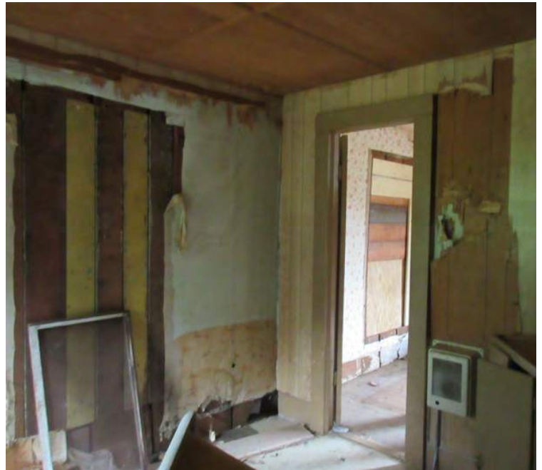
Figure 16: The image on the left depicts the southwestern corner of the original 1870's parlor. The wallpaper in this room is still intact apart from a strip (shown in this figure) that has been removed along the base of the walls in this room and the water damage that has occurred on the eastern wall (Figure 6). The image on the right depicts the removal of wallpaper in the original 1870's kitchen that displays the largest variety of underlying finishes out of all of the rooms in the house.
