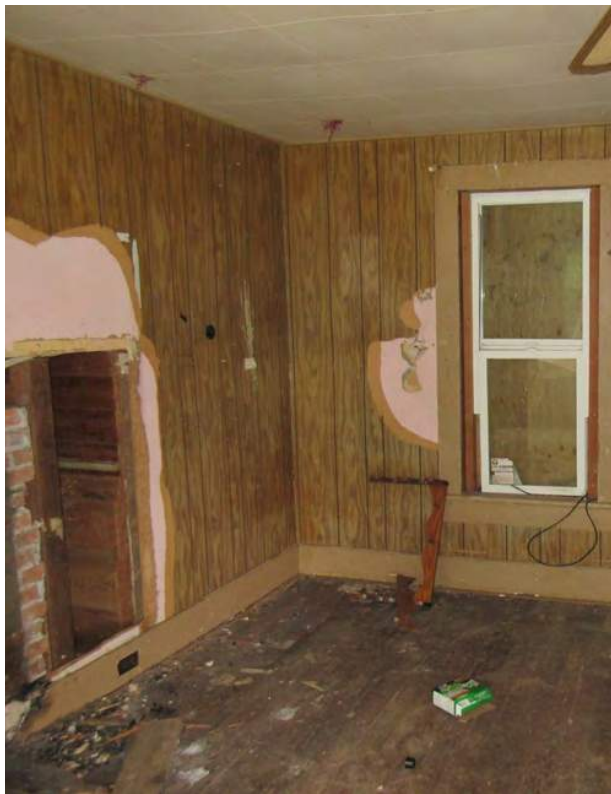
Figure 14: These images depict the living room in its current condition. Most pink wallpaper has been removed to reveal the underlying finishes, most notably around the fireplace. The final image depicts the damaged portion of the northern wall through which the dining room is visible on the other side.
