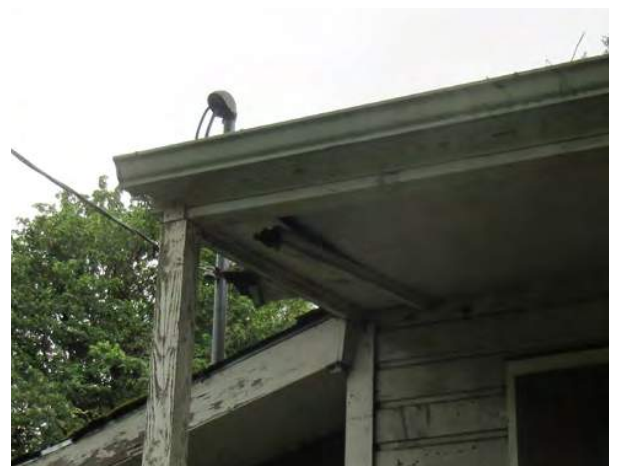
Figure 11: Both images above depict the southeastern corner of the current porch. The image on the left shows the paint erosion on the upper end of the post at this location, and the image on the right depicts the portion of the corner beam beneath this section of the roof that is missing.
