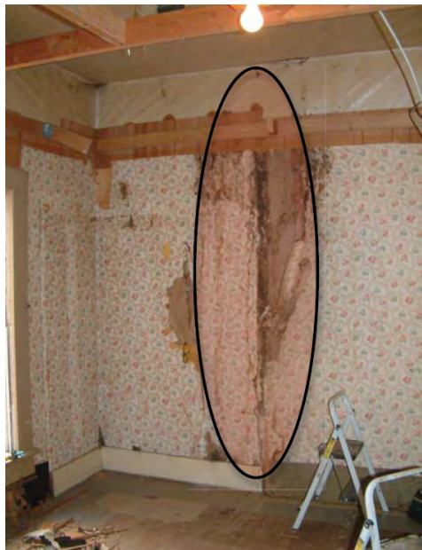
Figure 6: The image on the left is taken from the UO assessment and depicts the interior damage associated with the exterior northeastern critical area in 2010. The image on the right depicts how this damage has progressed over the past 7 years.
