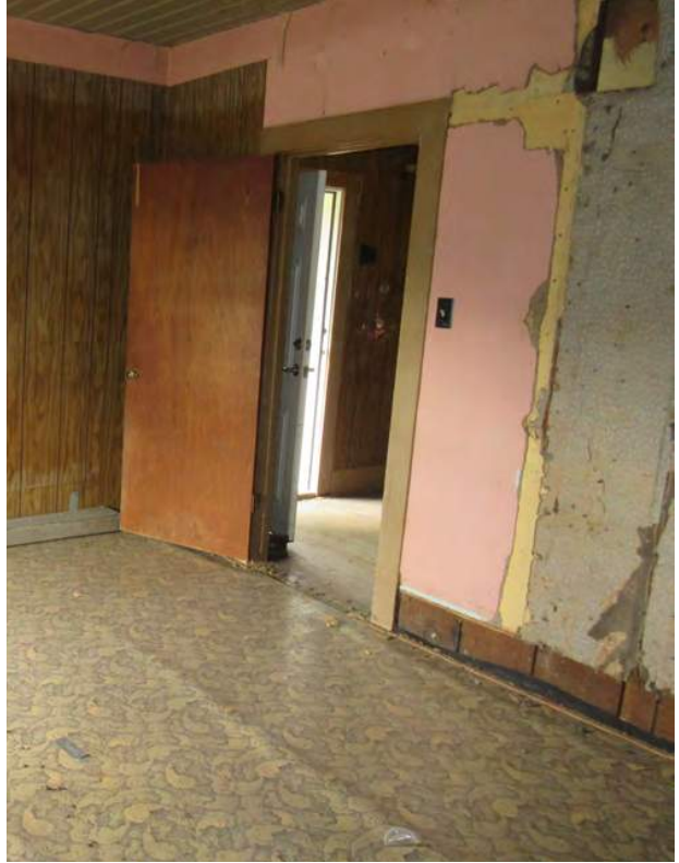
Figure 15: These images depict the current state of the dining room in the Briggs House. Most pink wallpaper from the walls and ceiling is missing, exposing the finishes beneath.
