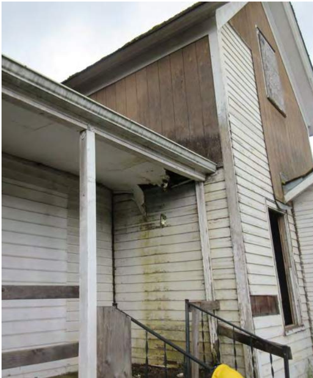
Figure 2: The image on the left (taken from the 2010 UO assessment) displays the roof above the porch in this northeastern critical area still intact, and the image on the right displays its current collapsed state. A piece of the cornerboard on the southeastern corner of the two-story structure (photo on the right) is missing on the northern face of the building.
