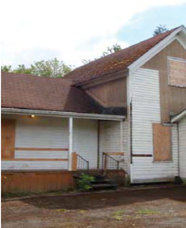
Figure 2: The image on the left (taken from the 2010 UO assessment) displays the roof above the porch in this northeastern critical area still intact, and the image on the right displays its current collapsed state. A piece of the cornerboard on the southeastern corner of the two-story structure (photo on the right) is missing on the northern face of the building.
