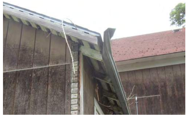
Figure 4 (left): The image above displays the tip of the cornice that is missing on the southern side of the two-story volume as well as the separation between the cornice and flashing on this edge. Figure 5 (right): This image depicts the loosely attached flashing on the southern roofline of the garage.
