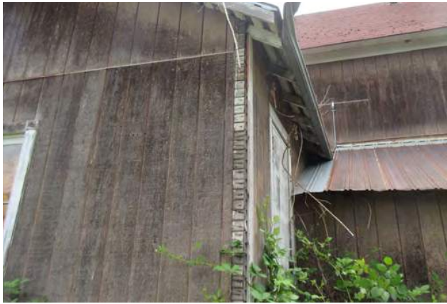
Figure 9: The image on the left displays the cornerboard that has been removed from the southeastern corner of the garage, and the image on the right displays the shiplap siding on this corner that shows paint erosion due to continuous water exposure over the past seven years.
