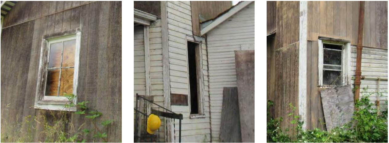
Figure 12: The three images above depict the splitting of the frames, muntins, and sills of the windows on the western façade of the garage and the northern and southern sides of the two-story upright structure, respectively.
