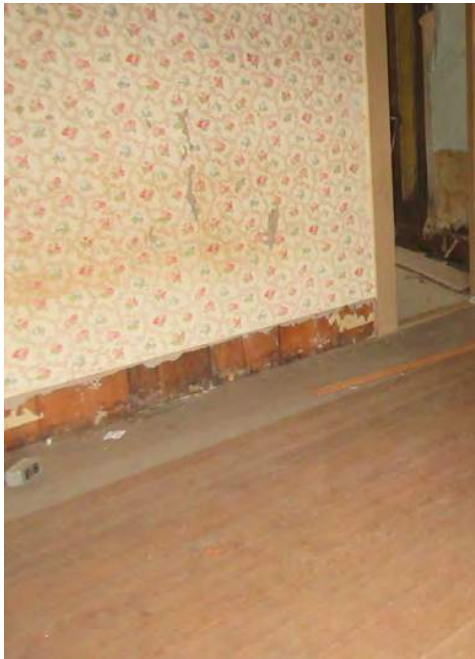
Figure 16: The image on the left depicts the southwestern corner of the original 1870's parlor. The wallpaper in this room is still intact apart from a strip (shown in this figure) that has been removed along the base of the walls in this room and the water damage that has occurred on the eastern wall (Figure 6). The image on the right depicts the removal of wallpaper in the original 1870's kitchen that displays the largest variety of underlying finishes out of all of the rooms in the house.
