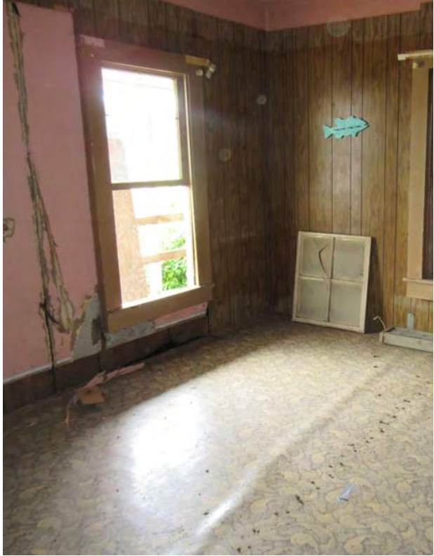
Figure 15: These images depict the current state of the dining room in the Briggs House. Most pink wallpaper from the walls and ceiling is missing, exposing the finishes beneath.
