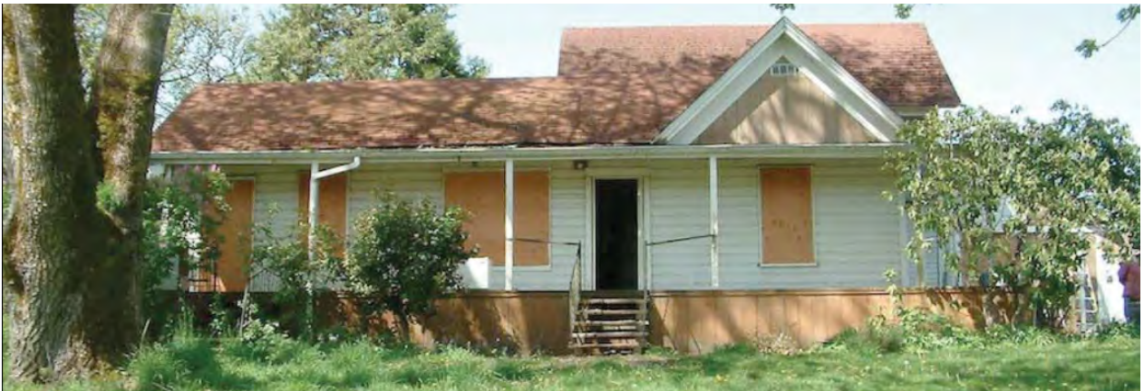
Figure 7: The image above exhibits a good example of the T-111 siding on the western façade of the main two-story volume and its attached shed that has accumulated water residue and lost a significant amount of color.
