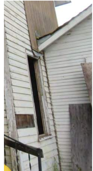
Figure 10: The first image above (left) exhibits the location where the cornerboard is missing at the juncture where the eastern façade of the garage meets the northern façade of the two-story structure. It also displays the paint chipping below the eave on the garage's eastern façade. The second image (right) depicts a close-up view of the vertical unpainted strip at the juncture along this eastern façade that suggests that a cornerboard had once existed there.
