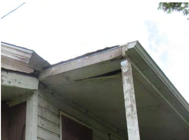
Figure 11: Both images above depict the southeastern corner of the current porch. The image on the left shows the paint erosion on the upper end of the post at this location, and the image on the right depicts the portion of the corner beam beneath this section of the roof that is missing.
