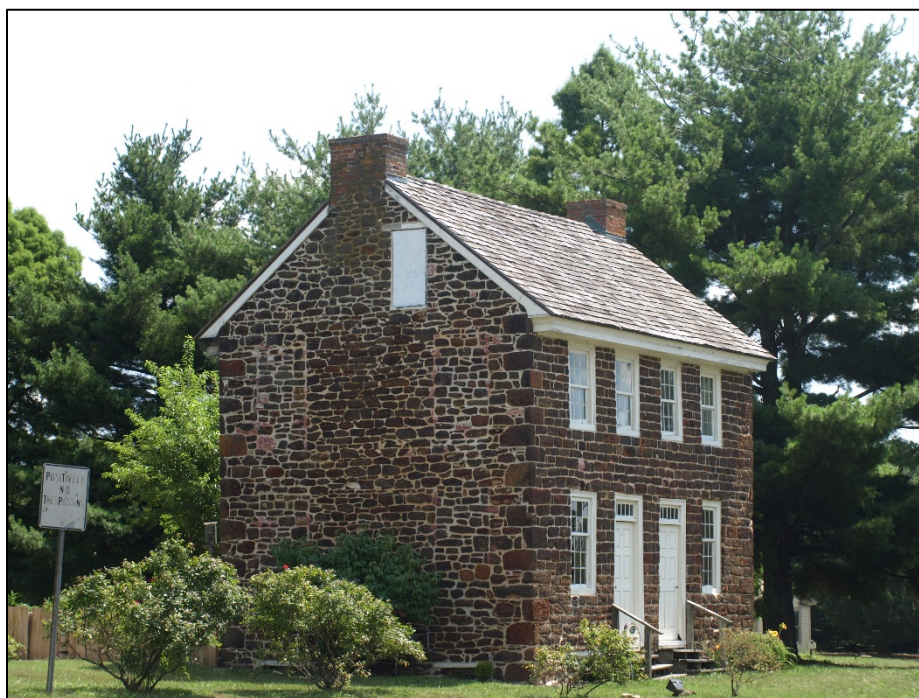
Figure 4. Old Stone House, Washington Township
