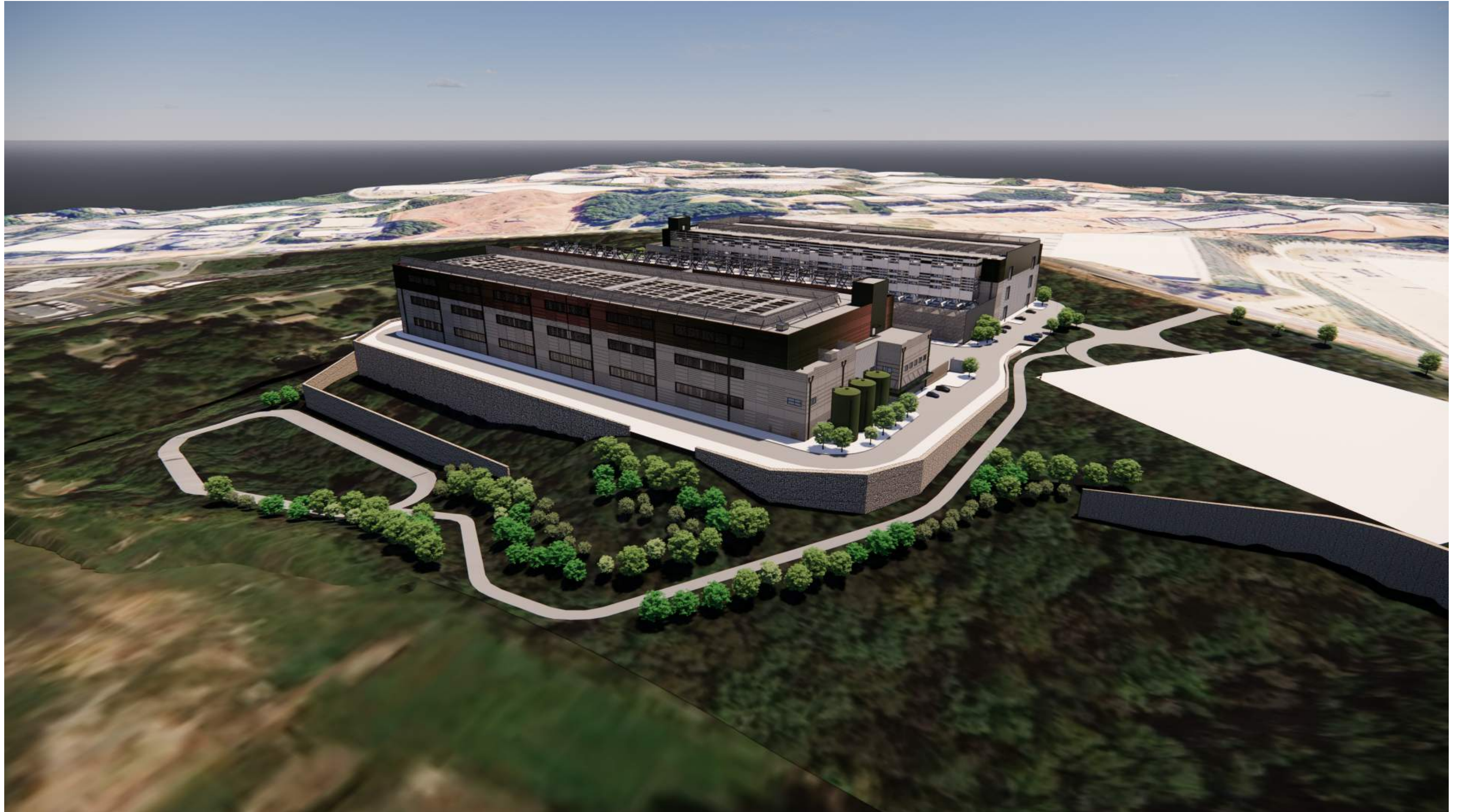
Aerial View Looking Northeast
