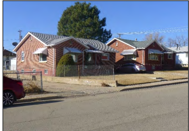
800 Block Atchison Ave, S side
