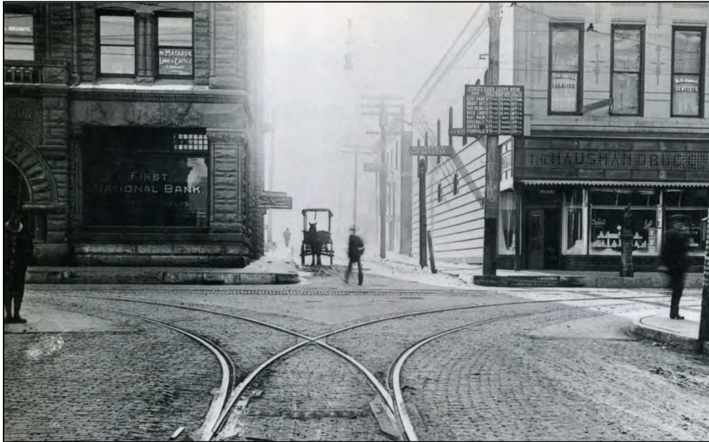
Figure 23. The brick paving and streetcar tracks at the intersection of Commercial and Main are shown in this early twentieth century image (view south). SOURCE: photograph, History Colorado, Denver, Colorado, in Fletcher, Centennial State Trolleys (1995), 156.
