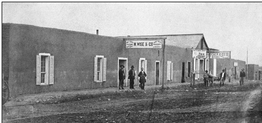
Figure 5. Many of Trinidad’s earliest buildings were one-story-flat-roofed adobes, as this 1868 view illustrates. SOURCE: Mangin, Colorado on Glass , 58.
