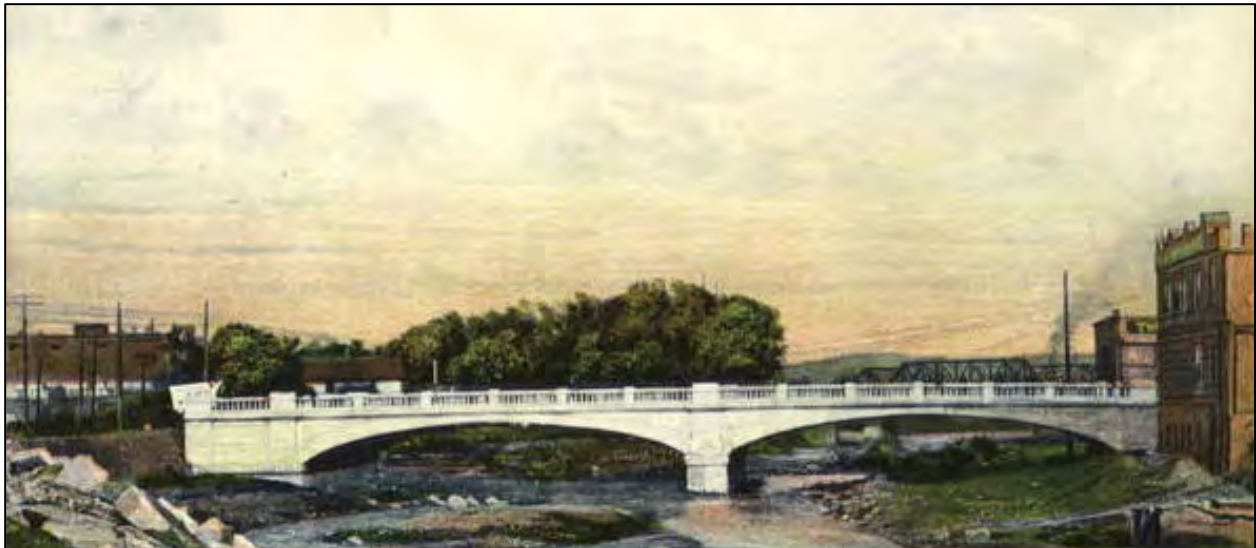
Figure 4. The Commercial Street Bridge over the Purgatoire River was demolished in 1990. SOURCE: Historic postcard view, Tom and Laurie Simmons, historic postcard image collection, Denver, Colorado.
