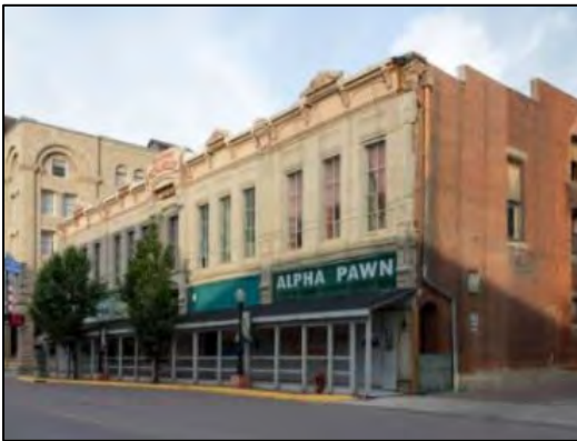
Jaffa Opera House, Hausman Drug, 5LA.2181, 100-116 W. Main St, National Register listed 1972 (within Corazon)
