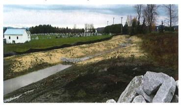
ceived. A notice to proceed to was issued to Hebert Excavation on October 5. The contractor started work promptly. The contract includes filling and stabilizing an eroded bank at the edge of the woods behind St. Sylvester Cemetery; improving the swale from the rec area with a wider, flatter bottom and stone check dams; constructing a bioretention basin; and building a level lip spreader pole inventory is being conducted in five municipalities and is for
