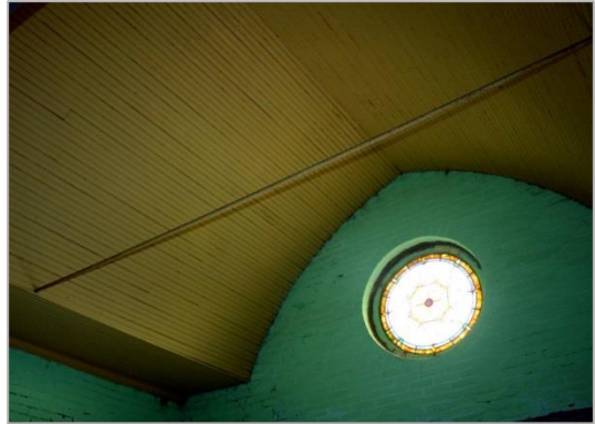
Looking back towards the entry door, the 33 inch wide shoulder at the ceiling can be seen as well as the arched ceiling. The stabilizer rod spans the interior.
