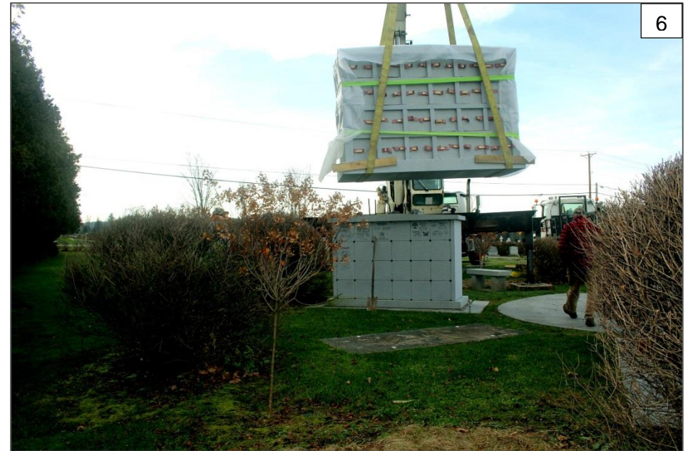
Photo 5: the crane operator swung the columbarium over the existing park. The contractor added boards at the base of the unit to keep the straps off of the granite base. Photo 6: the crane operator brings the columbarium closer to the existing concrete foundation. Photo 7: Joe and Vinny Calcagni of GCB guided the columbarium as it came down to ensure an even placement on the existing foundation. Photo 8: Mr. Garceau noticed the end of the unit facing the center of the circle did not have the unit number visible, the heavy plastic made it difficult to see them. The contractor spun the unit around to display the numbers.
