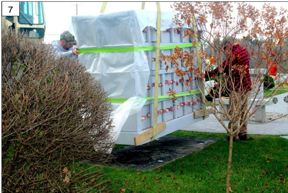
Photo 5: the crane operator swung the columbarium over the existing park. The contractor added boards at the base of the unit to keep the straps off of the granite base. Photo 6: the crane operator brings the columbarium closer to the existing concrete foundation. Photo 7: Joe and Vinny Calcagni of GCB guided the columbarium as it came down to ensure an even placement on the existing foundation. Photo 8: Mr. Garceau noticed the end of the unit facing the center of the circle did not have the unit number visible, the heavy plastic made it difficult to see them. The contractor spun the unit around to display the numbers.
