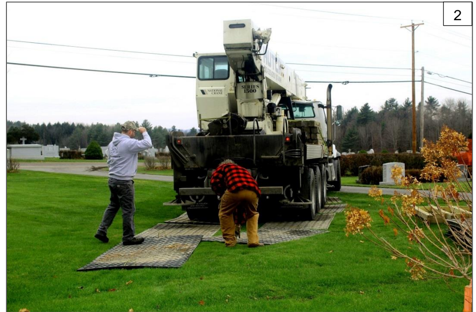
Photos taken 17 November 2023. Photo 1: Direct from the factory floor, the shutters have been braced with wood wedges and untreated building paper to keep them in place during transit over the rough roads. Photo 2: GCB Corp. did the work to set the columbarium. They spread out some hard rubber planking to help save the lawn from the heavy loads. Photo 3: a two-truck process, the one on the left brought the columbarium to the cemetery, the one on the right brought the heavy duty crane. Photo 4: With the two trucks in place, strap loops hanging from the hook on the end of the crane boom were slipped under the columbarium and it was lifted off of the truck. As seen in Photo 1, the columbarium traveled on blocks set on the bottom of the truck for easy strap placement.
