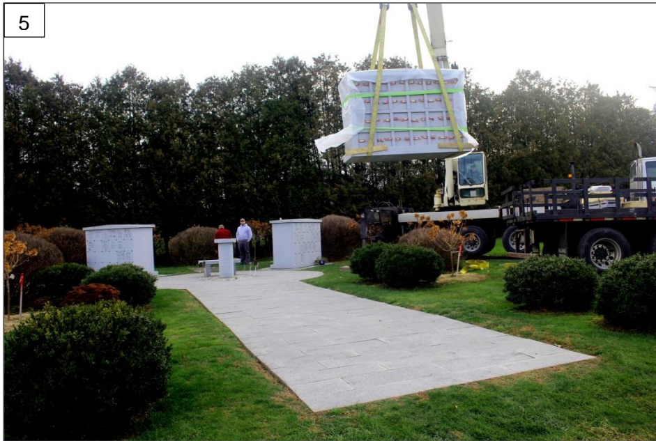
Photo 5: the crane operator swung the columbarium over the existing park. The contractor added boards at the base of the unit to keep the straps off of the granite base. Photo 6: the crane operator brings the columbarium closer to the existing concrete foundation. Photo 7: Joe and Vinny Calcagni of GCB guided the columbarium as it came down to ensure an even placement on the existing foundation. Photo 8: Mr. Garceau noticed the end of the unit facing the center of the circle did not have the unit number visible, the heavy plastic made it difficult to see them. The contractor spun the unit around to display the numbers.
