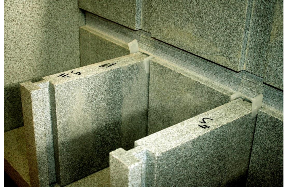
Above: The parts and pieces that make up the niches are held in place using some kind of epoxy and small plastic wedges while the epoxy dries. Below: an organized pile of parts and pieces awaiting assembly. Note the numbers on the individual pieces, these numbers correspond to those shown on the shop drawings provided to the cemetery commission.
