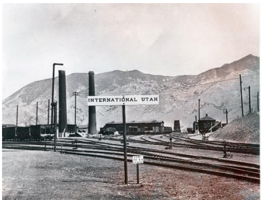
Railroad Entrance into the International Smelter, Tooele Valley Museum Collection
