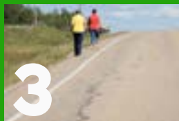
Lack of Sidewalks
