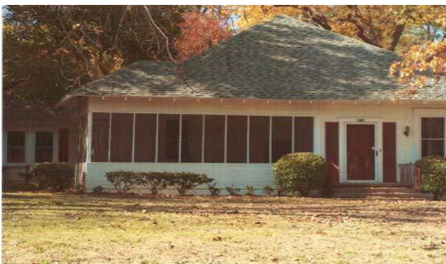
When a porch is enclosed or screened, it shall be done with a clear transparent material. This material should be placed behind porch columns.
