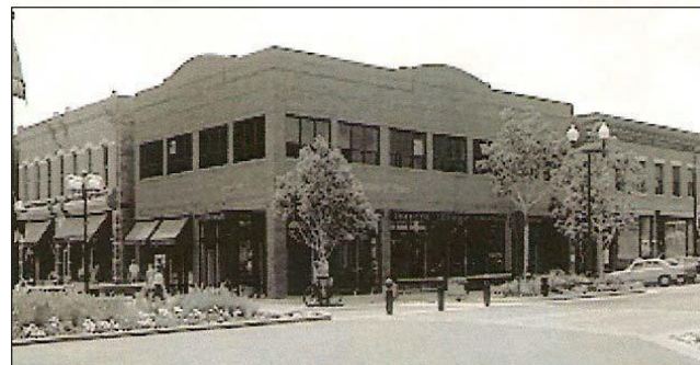
After: Simplified interpretations of traditional building elements, including a transparent first floor with display windows and an ornamental cornice, help this new building fit into its context.
