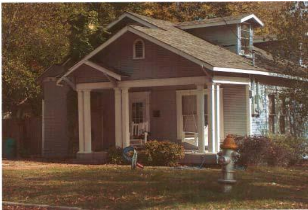
When replacing porch posts, use supports that are of adequate size. This porch reconstruction was based on neighboring houses of similar character and age.
