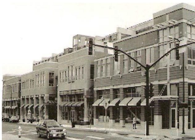
This single infill building is divided into smaller building modules that reflect traditional building widths. Upper floors step back from the front, thus maintaining the traditional two-story scale of the street.
