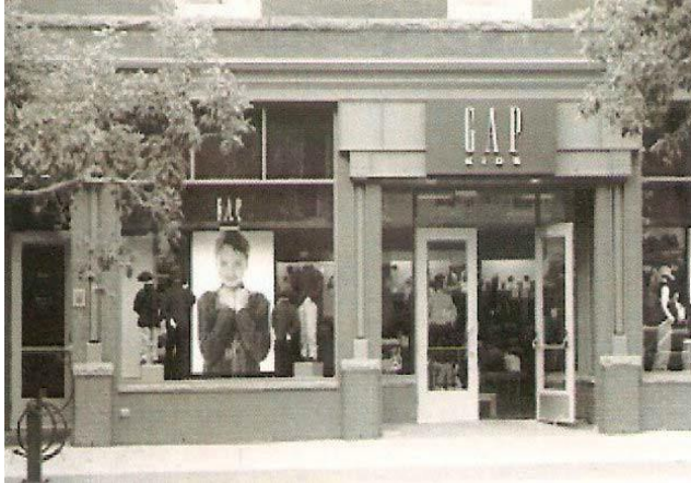
If evidence of the original design is missing, use a simplified interpretation of similar storefronts. The storefront still should be designed to provide interest to pedestrians.
