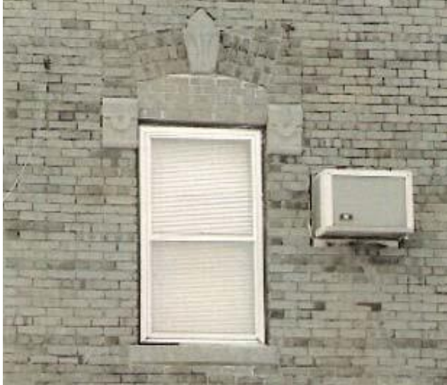
Do not locate window air conditioning units on a building's primary facade.
