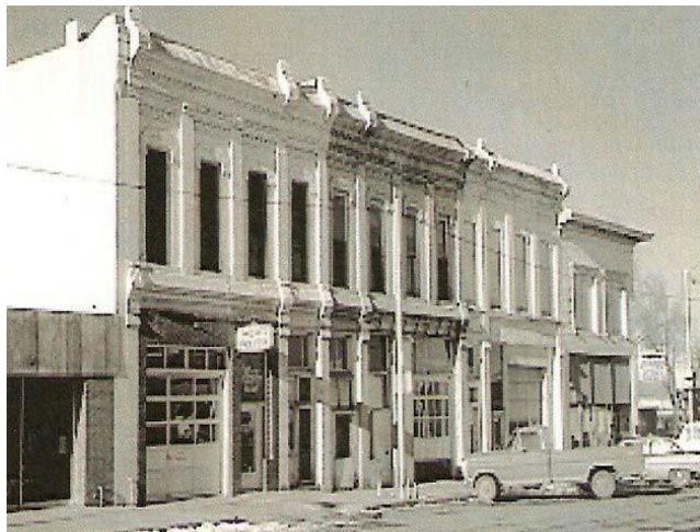
This row of buildings had lost some details over time and a monochromatic color scheme obscures the original design character. Overhead garage doors that had replaced original storefronts were later alterations without historic significance. (Compare with the “after” photograph below.)
