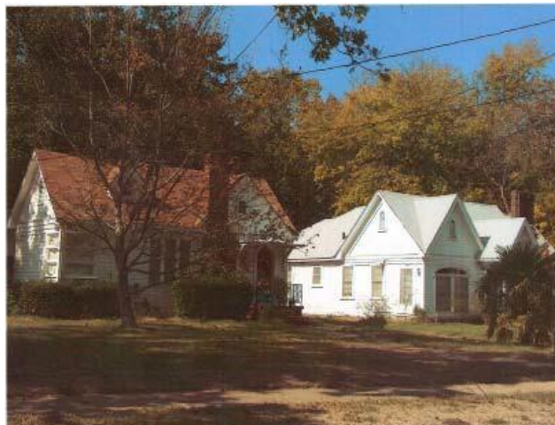
In residential areas, most roof forms are pitched, such as gabled and hipped.
