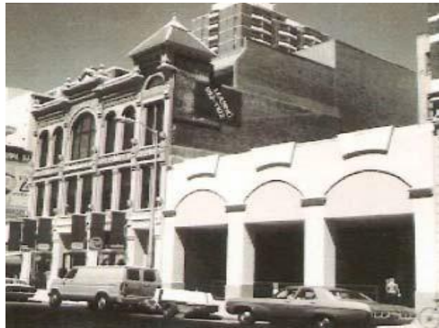
In the angle view above, two newer floors are visible. Note how in this building the addition cannot be seen when looking at the building straight on in the top photo.
