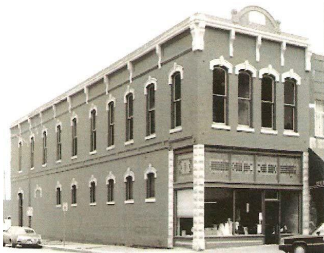
On a commercial building, first floors should be more transparent than upper floors. Upper floors should appear more solid than first floors.
