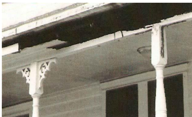
Replace missing original details in kind.
