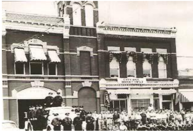
Using historic photographs can help in determining the original character. (Compare with below.)
