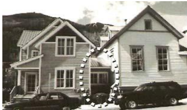
Design an addition to be compatible in size and scale to the main building. This addition appears to be in scale with the original building because it is separated with a smaller connecting structure
