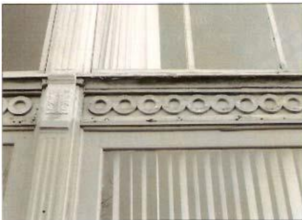
Protect wood features from deterioration.
