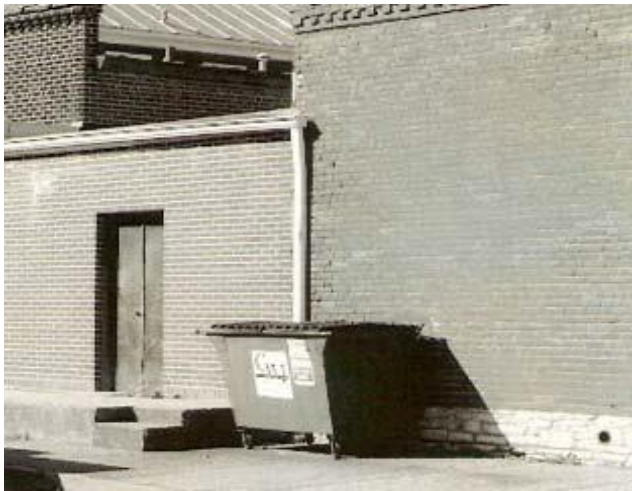
Trash areas, including large waste containers or dumpsters, should also be screened from view, using a fence, hedge or enclosure.
