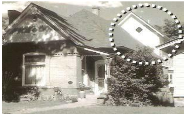
An addition shall be set back from any primary, character-defining facade. An addition should be to the rear of the building, when feasible.
