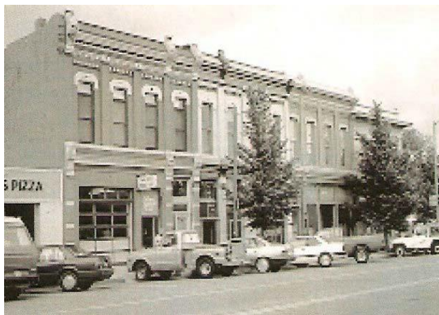
After rehabilitation, the row of buildings shown in the photograph above conveys a stronger sense of its historic character. Note that some old uses were retained, while other new uses were also introduced. Some noncontributing alterations were removed and storefronts reconstructed. One was retained, but was painted to minimize impacts.
