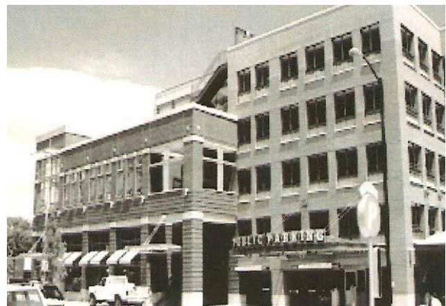
A part of this infill building is a parking structure that is set back from the front and sides of a retail wrap. The openings in the parking section reflect window proportions similar to those seen historically in the area.
