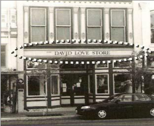
When utilizing the sign frieze as the sign placement location, it is important to respect the frieze borders.
