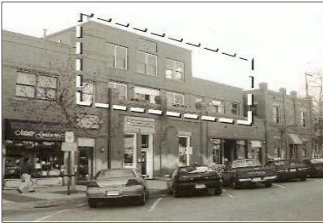
An addition should be set back from the primary, character-defining facade, to preserve the perception of the historic scale of the building.
