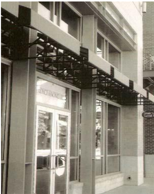
A new commercial store front building should incorporate display windows, transom window, a kickplate and recessed entry.
