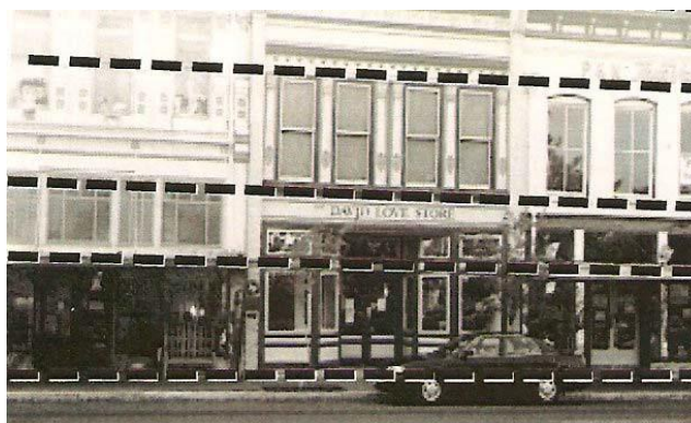
A building shall maintain the alignment of horizontal elements along the block.
