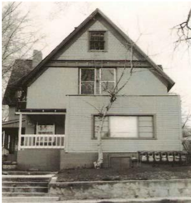
Design a new addition such that the original character can be clearly seen. This addition to the front of the historic structure is inappropriate.
