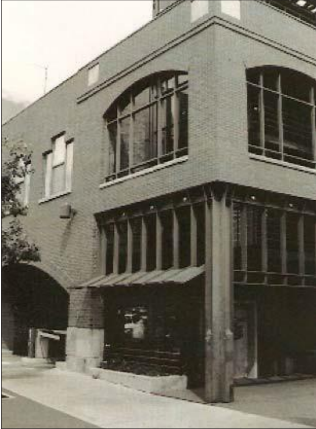
This parking structure incorporates a wrap of retail stores along the street edge. The storefronts are contemporary interpretations of the historic downtown context.
