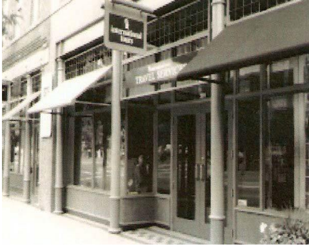
Contemporary interpretations of traditional building elements are encouraged. In this case, shed form awnings are stretched across rigid frames. Transom windows are expressed with a metal grill design.
