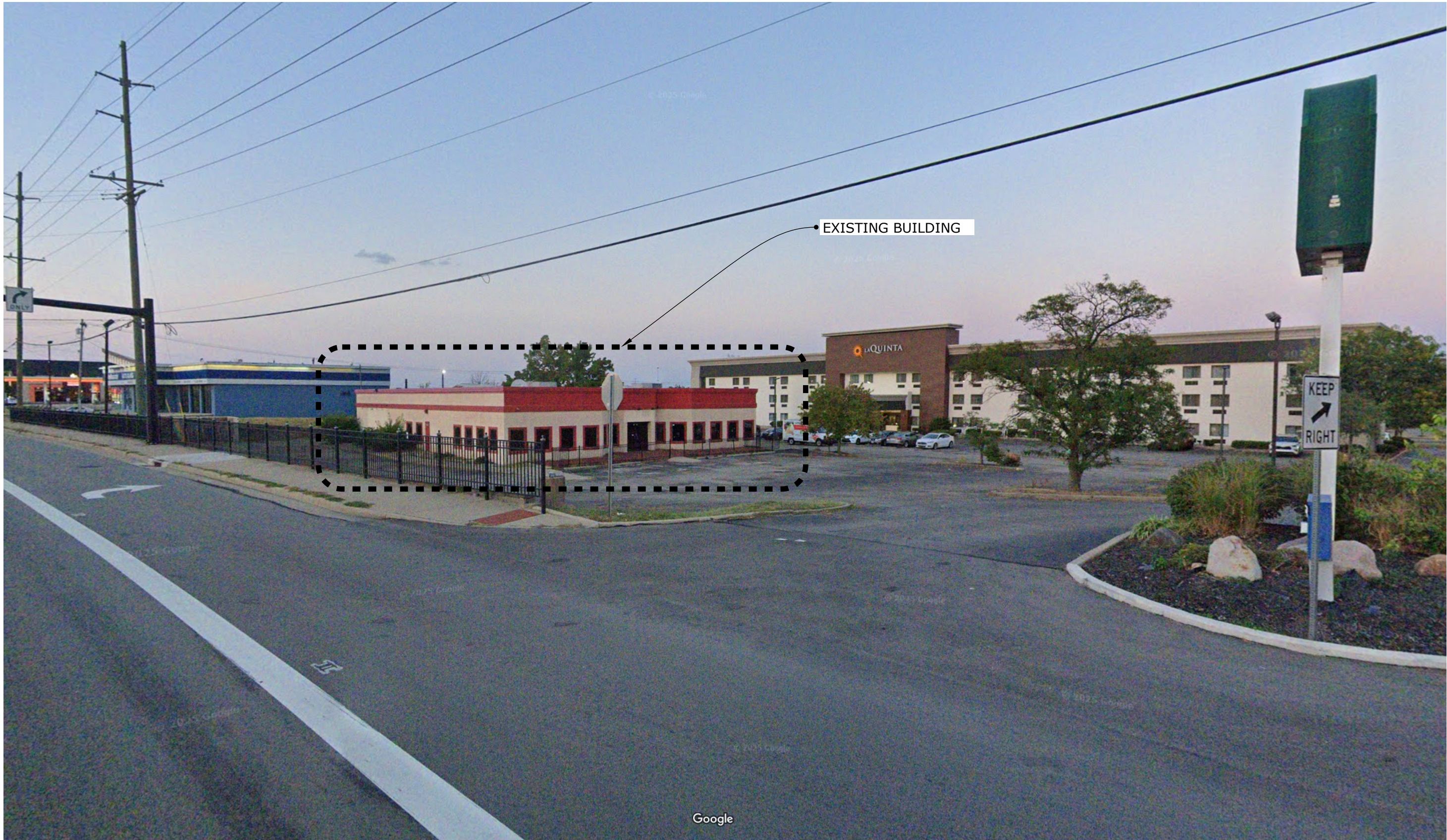
EXISTING BUILDING SITE
