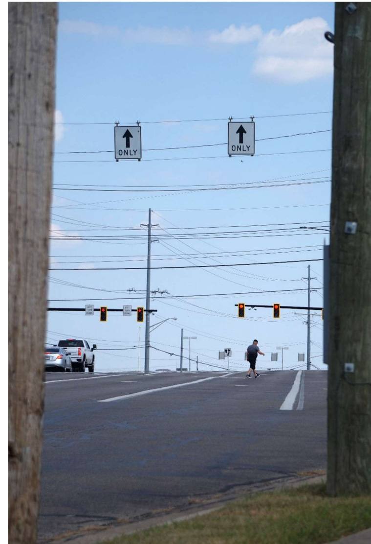
Figure 21: A VRU crossing W Kemper Rd at Princeton Pike.
