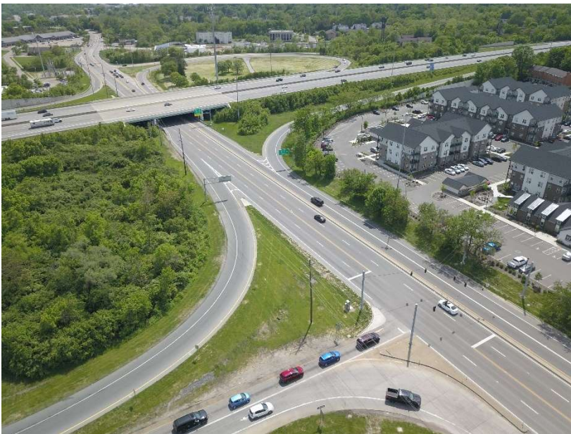
Figure 32: Springfield Pike & I-275 ramps.
