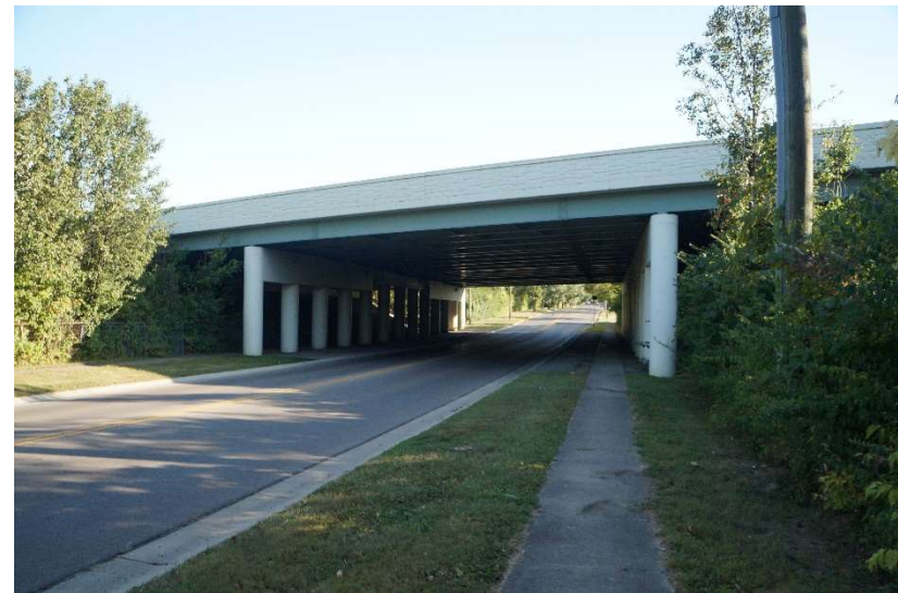
Figure 6: I-275 Bridge over Kenn Rd.
