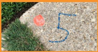
They identify areas marked by Town staff as potential tripping hazards and are scheduled to be repaired by a company called Precision Concrete Cutting.
