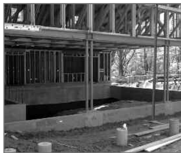
View of New Covered Pavilion Area.
