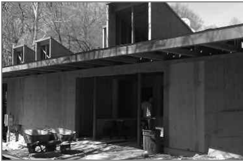
New Pool Entrance Under Construction
