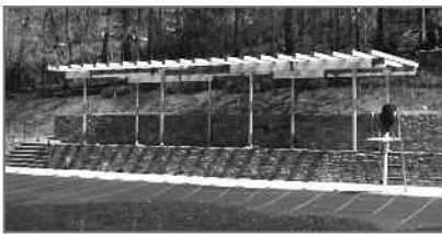
New Shade Structure Along Widened West Terrace.
