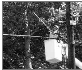
Pepco – Tree Trimming
