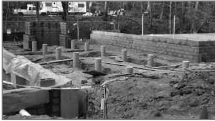
Piers for the New Deck that Adjoins the Grill Area Next to the Pavilion.
