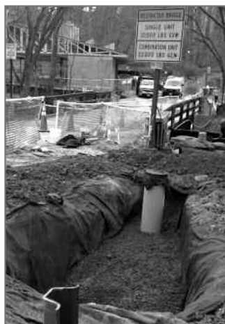
Construction of One of 3 Bio-Retention Facilities to Manage Storm Water Runoff.
