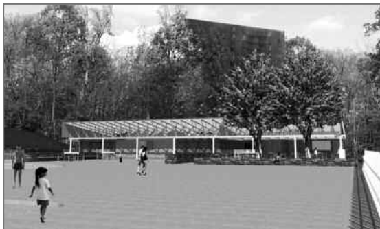
Somerset Pool Facility Renovation Project.
