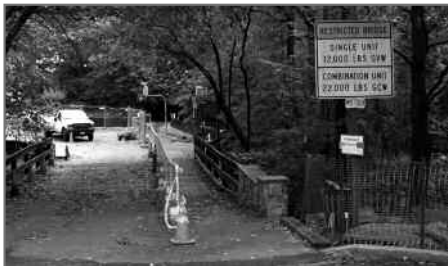
Construction Fencing and a Pedestrian Walkway Installed.
