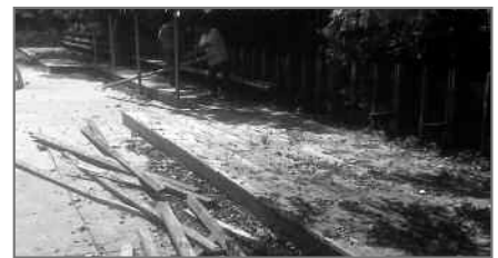
Removing Some Pool Decking to Increase Setback from the Stream.
