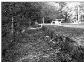
Removal of the Old Wood Extension from the Deck Will Make Room for Planting More Indigenous Trees and Shrubs to Help Retain the Stream Bank.
