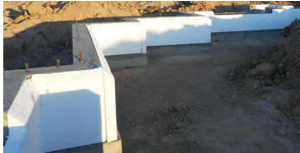
EPS placement in a frost-protected shallow foundation
