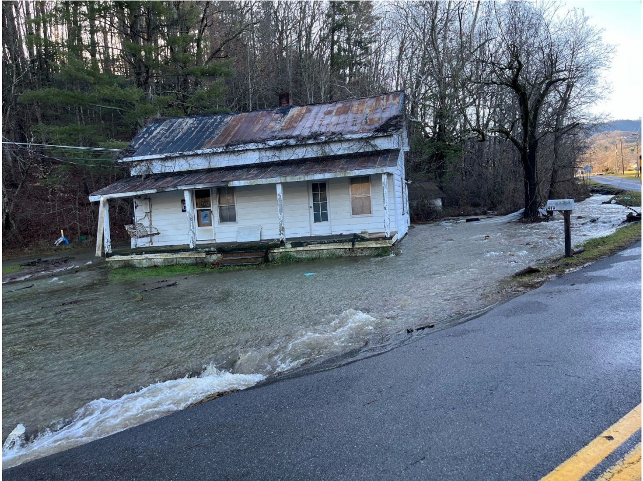
Photos of Old St. Clair's Creek flooding:
