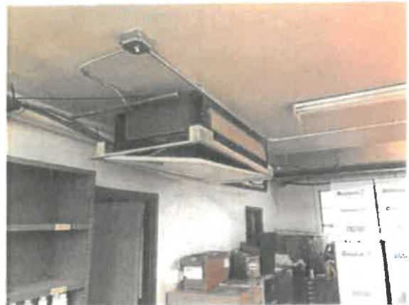
Existing cooling fan coil unit.
