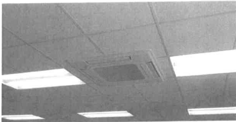
VRF ceiling cassette heating and cooling air handler.
