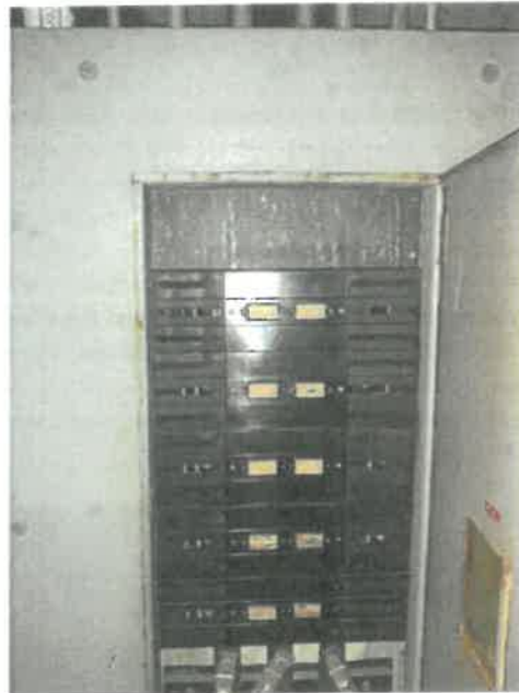
Original attic panel board and exposed bus.
