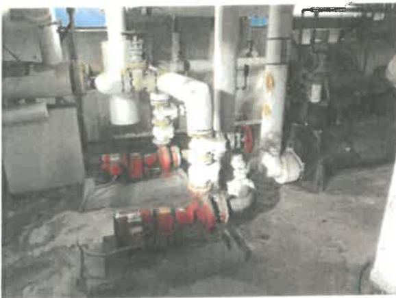
Existing water-cooled chiller and water pumps.
