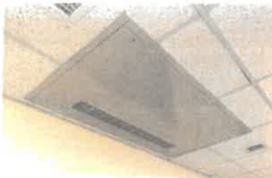
New heating and cooling fan coil unit.
