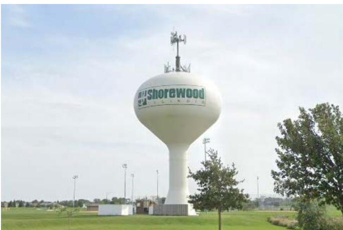
Elevated tank at Walnut Trails. Image Credit | B&W
