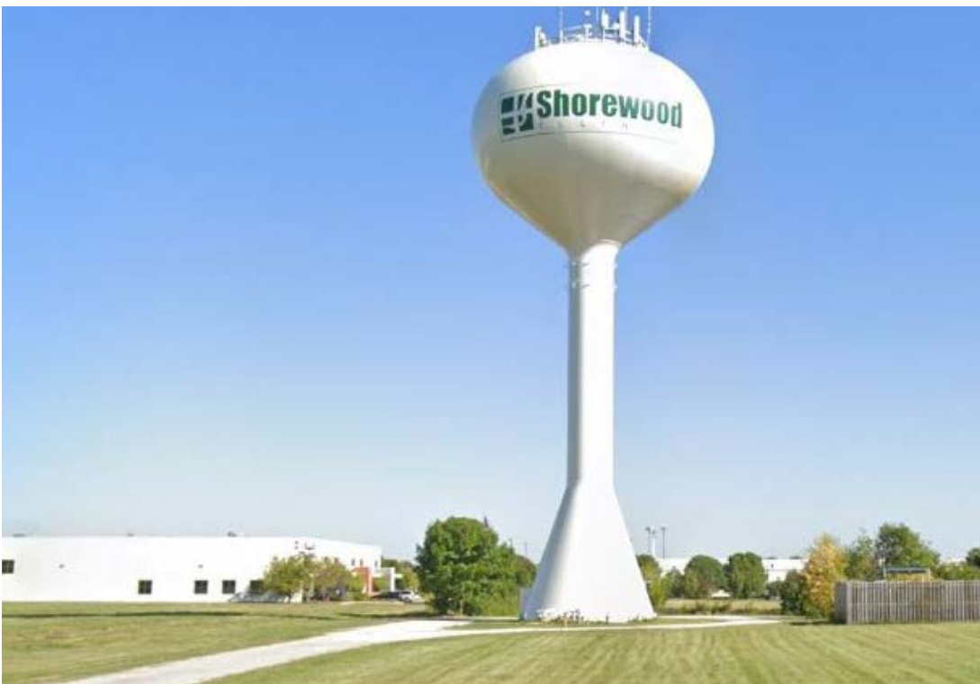
Elevated storage tank at Mound Rd. Image Credit | B&W
