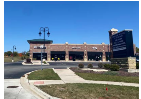
Small commercial complex on Jefferson St. & Brook Forest Ave.
