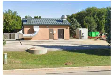
Pump Station on Black Rd Image Credit | Baxter & Woodman
