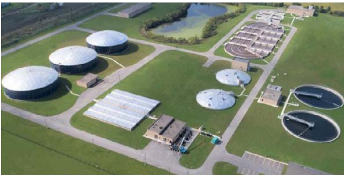
Joliet Aux Sable WWTP. Image Credit | B&W
