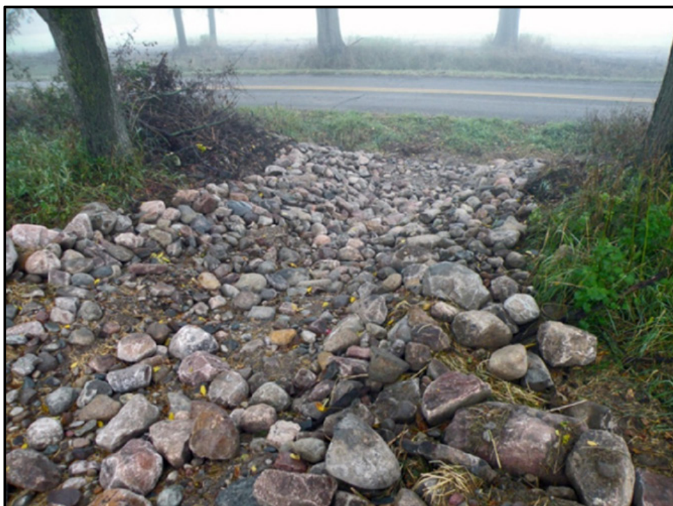
Figure G.19. Example of a grade stabilizer.
