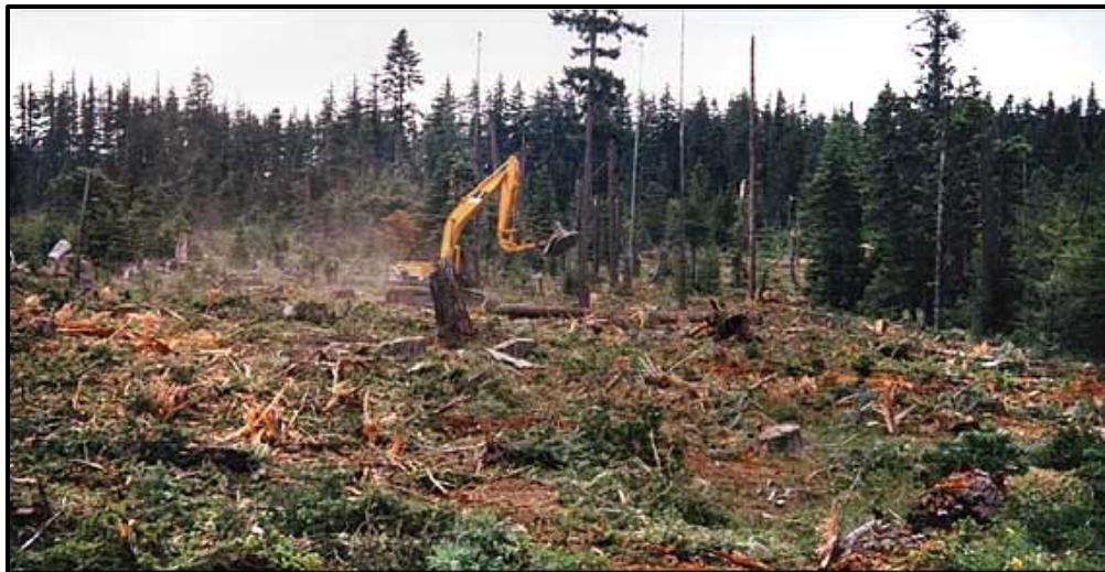
Figure G.9. Mechanical slashing and spreading of vegetation.
