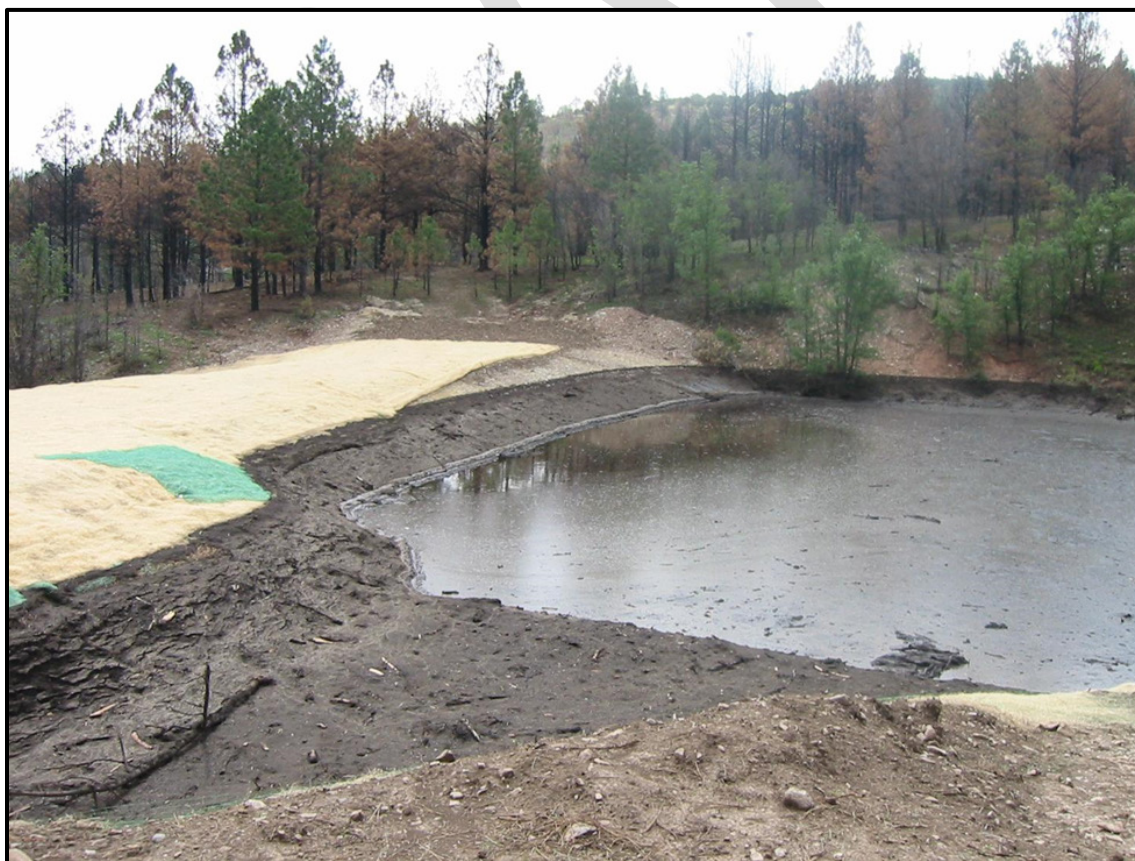
Figure G.17. Example of a debris basin.
