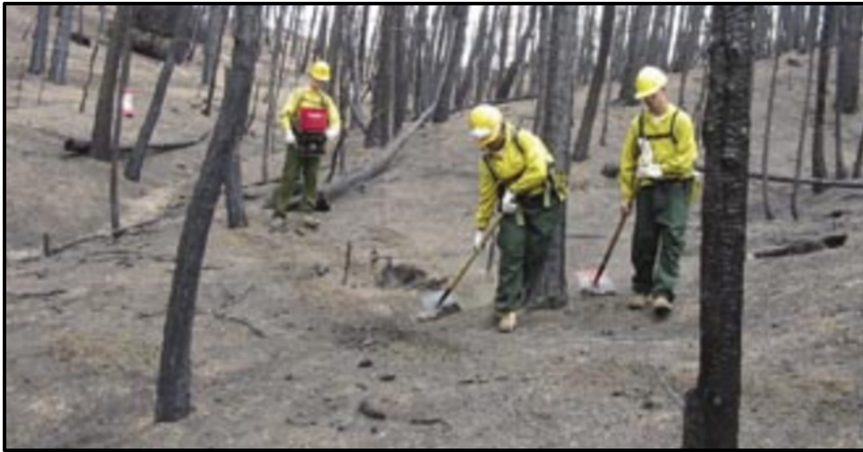
Figure G.14. Crews scarify soil in a burn area by hand.
