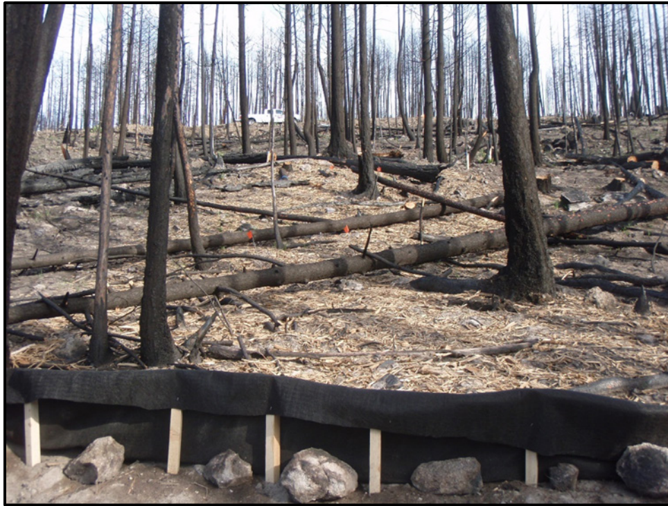
Figure G.13. Silt fence constructed at the bottom of a slope post-fire. Contour felled logs can be seen uphill from the fencing as well.
