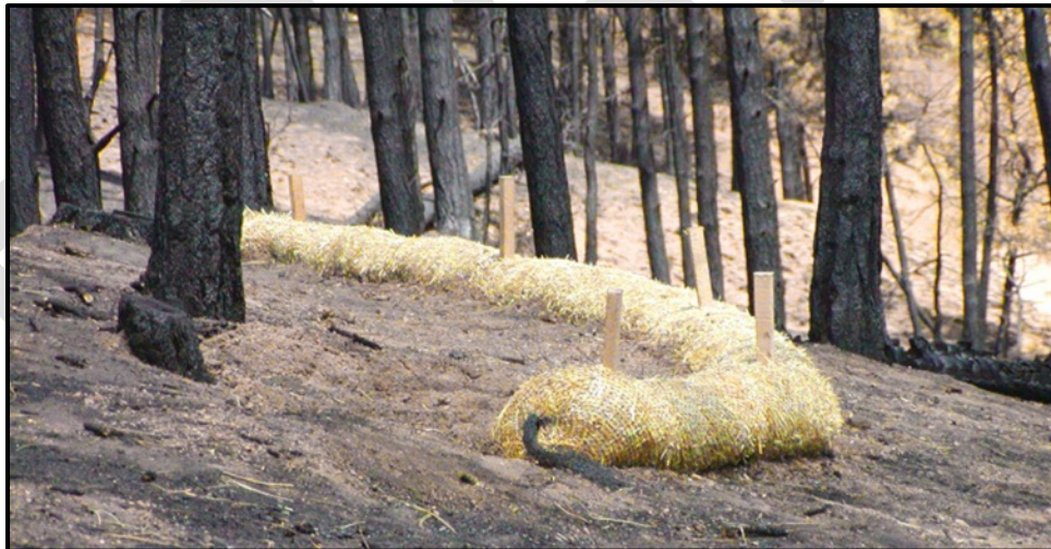
Figure G.11. Fiber rolls in place on a hillslope following a fire.
