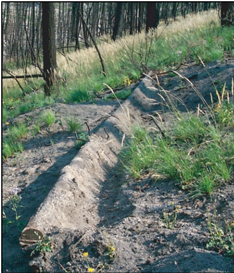
Figure G.7. Log erosion barrier.
