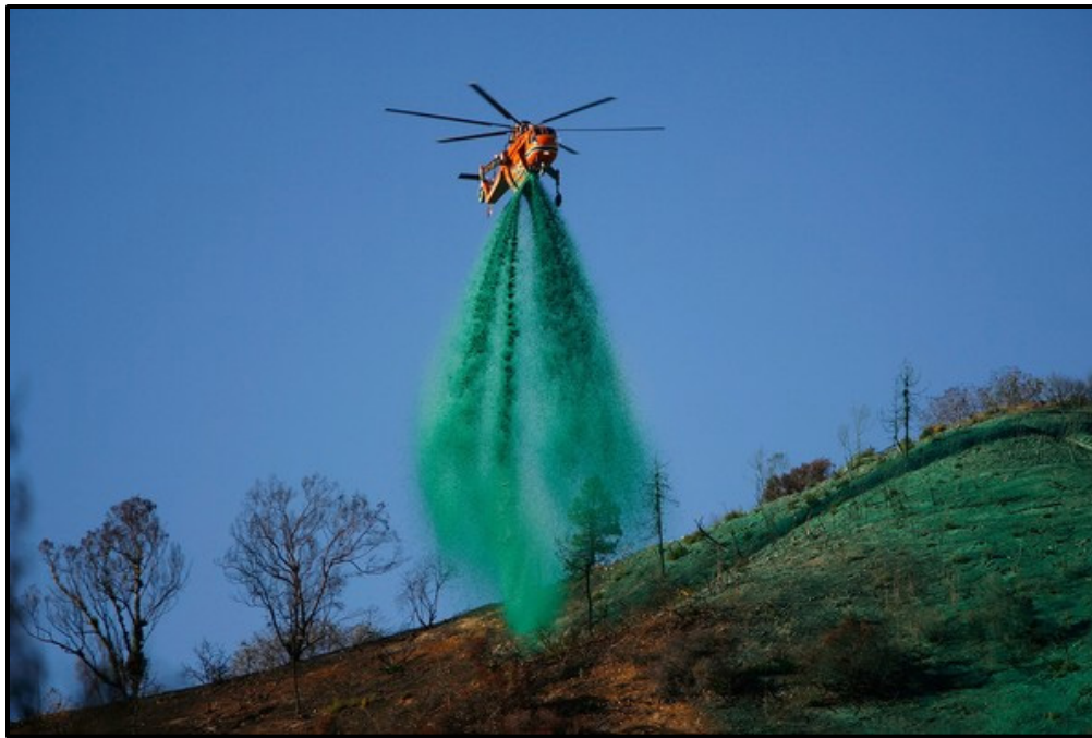
Figure G.6. Hydromulching via aerial delivery on a slope.
