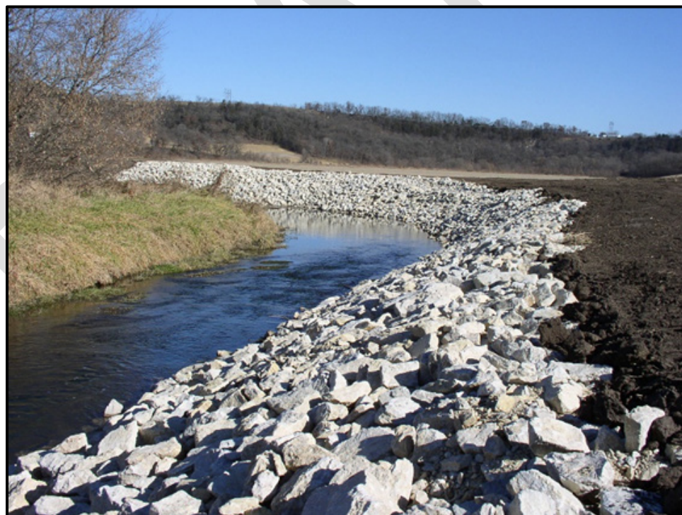
Figure G.27. Example of stream bank armoring.
