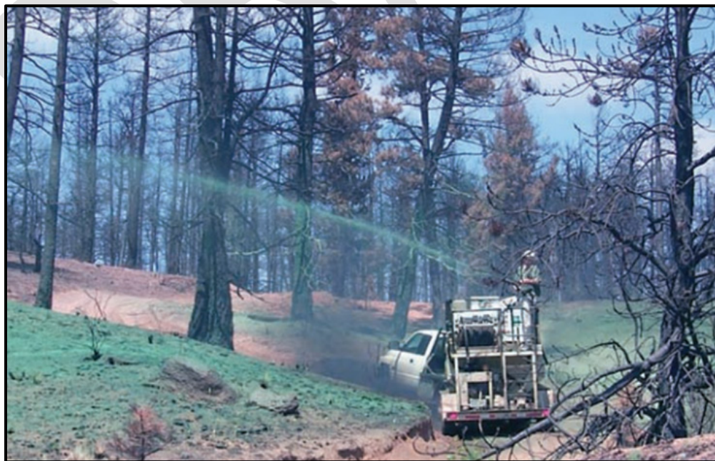
Figure G.5. Post-wildfire hydromulching operations using a hydroseeder trailer.
