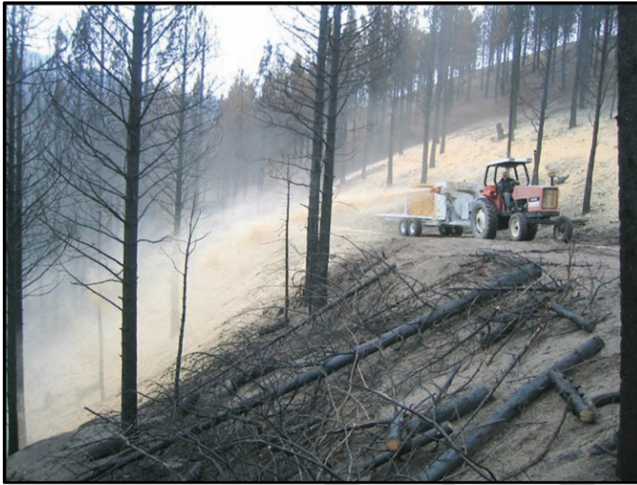
Figure G.1. Dry mulch being mechanically applied to a hillslope.
