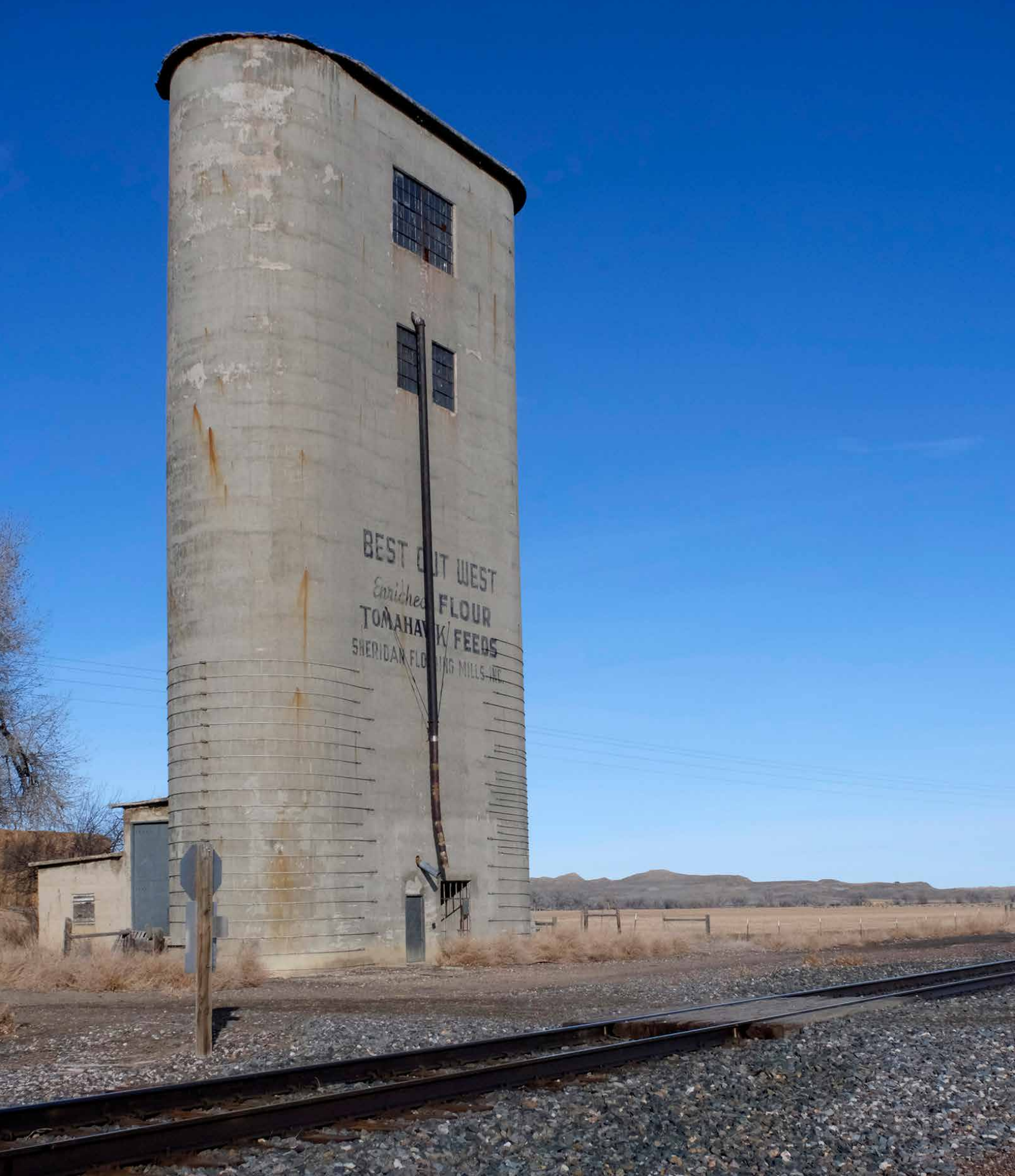
Silo in Leiter, Wyoming. Photo Courtesy of Sheridan Community Land Trust
