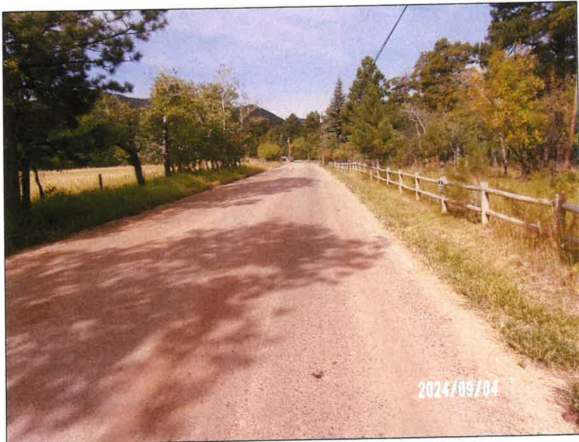
Fig 3 North Piny Rd looking west (subject parcel on right)
