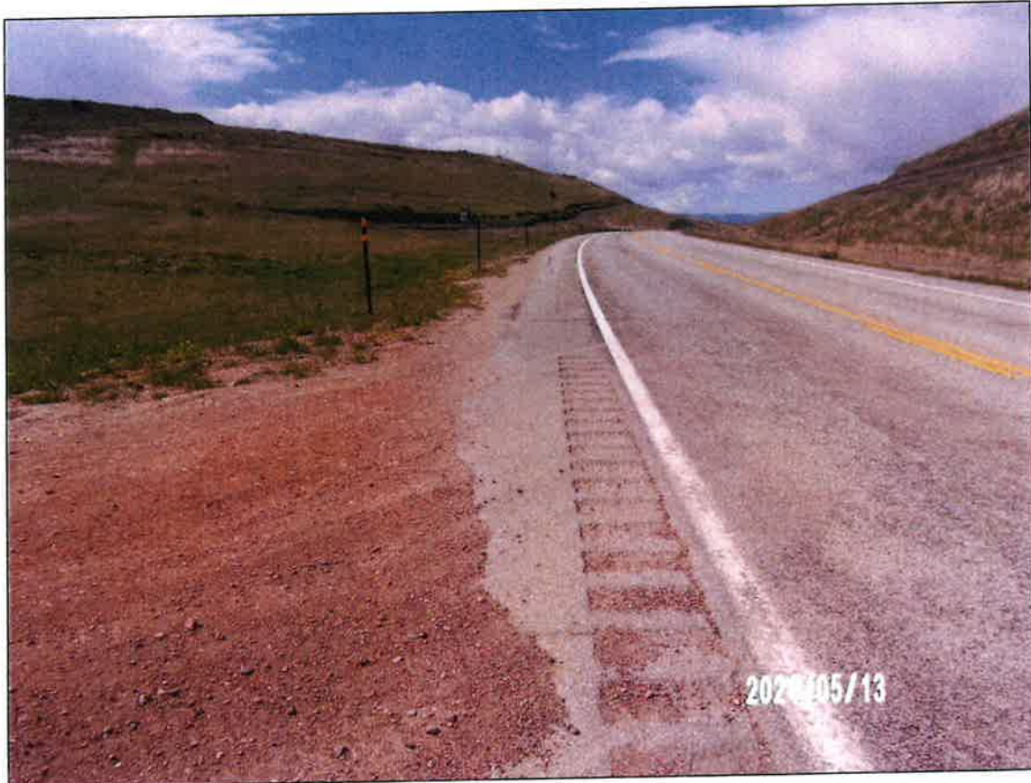
Fig 4 State Hwy 338 (looking west from Bree Lynn Rd access)
