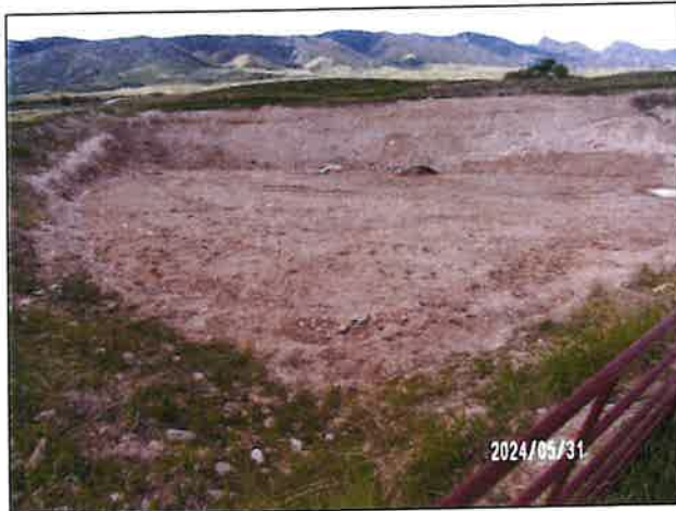
Fig 1 Existing Husske Quarry (looking west)
