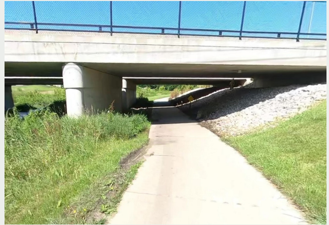
The Little Walnut Creek Trail going between a pier (on the left) and abutment (on the right) of the 156th Street bridge in Urbandale, IA
