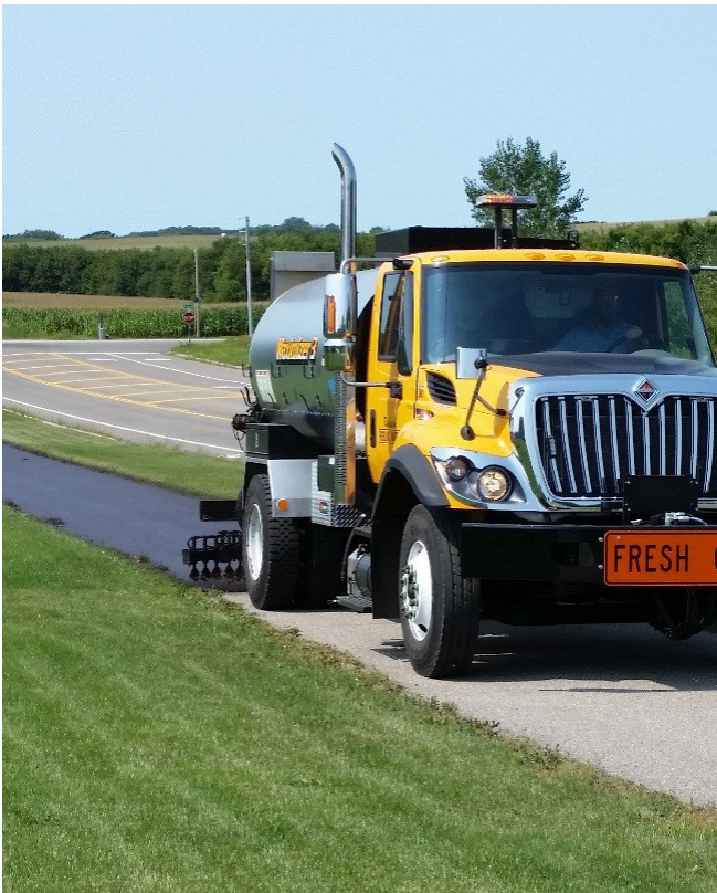
FIGURE 3.26 Fog sealing asphalt trails prevents costly, premature trail reconstruction projects. Credit: City of Rochester, MN
