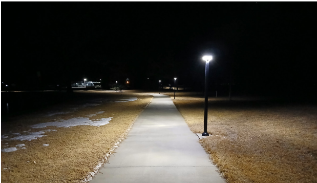
FIGURE 4.3 Pedestrian scale lighting along a trail in Tyndall, SD.
