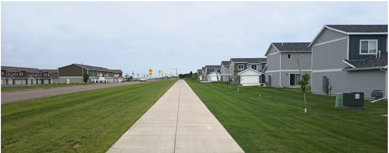
FIGURE 3.4 The Willow Street trail along the north side of the road is 10' wide and concrete.
