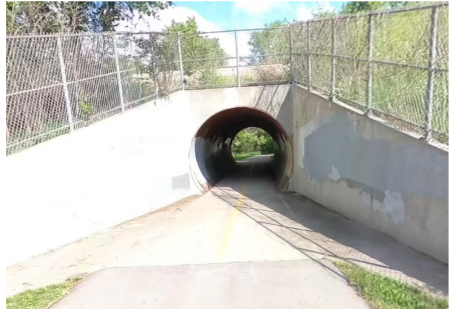
The Vern Willey II Trail going through a culvert pipe under a railroad in Altoona, IA
