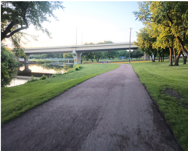
FIGURE 3.22 The Sioux Falls Recreation Trail as it passes under the E 26th Street bridge.
