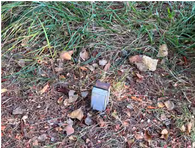
Figure 17: Non-functional outlet at Amphitheater limits utility
