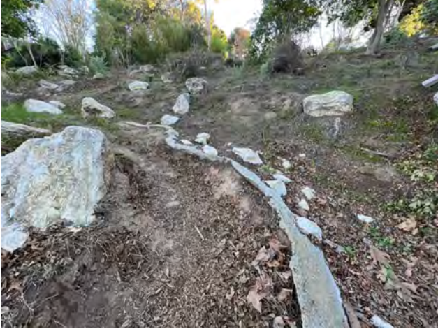
Figure 12: Exposed gunite from old stream bed at lower pond
