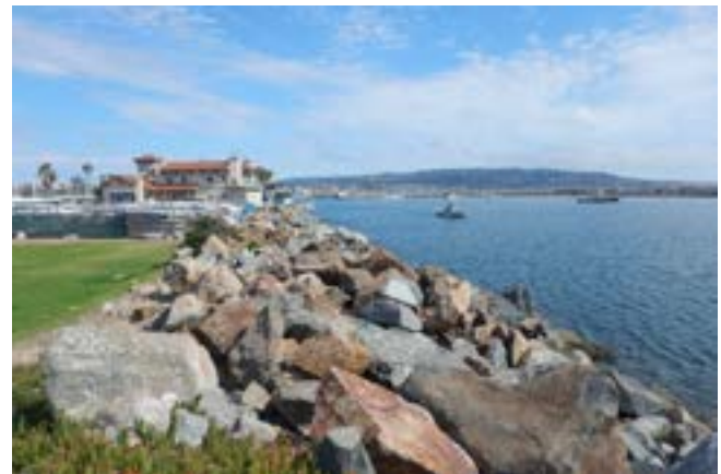
Mole B rock revetment
