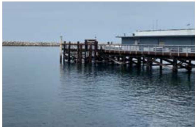
Existing infrastructure of Sportfishing Pier
