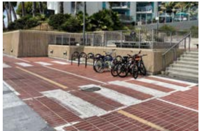
Bike path at upper deck of International Boardwalk
