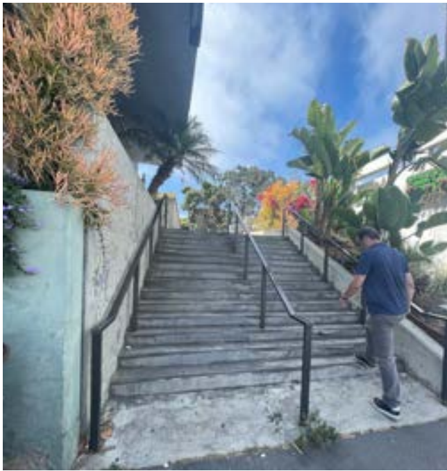
Stair at the north end of International Boardwalk
