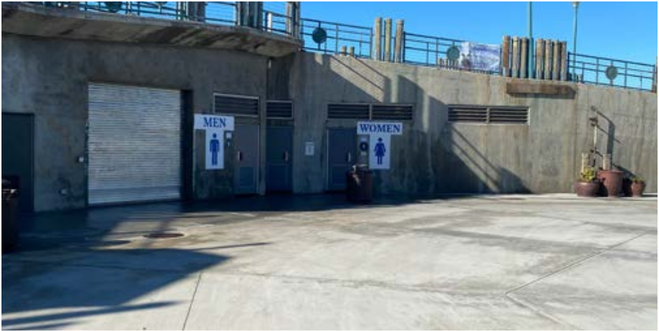
International Boardwalk Public Restrooms near courtyard
