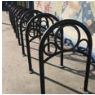
Repainting existing bike racks
