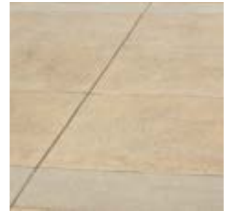
Smooth warmer concrete
