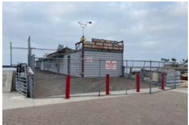
Entrance to the pier
