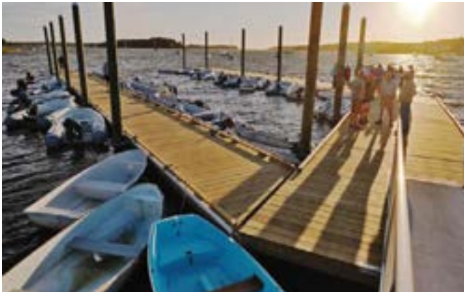
Timber dinghy dock
