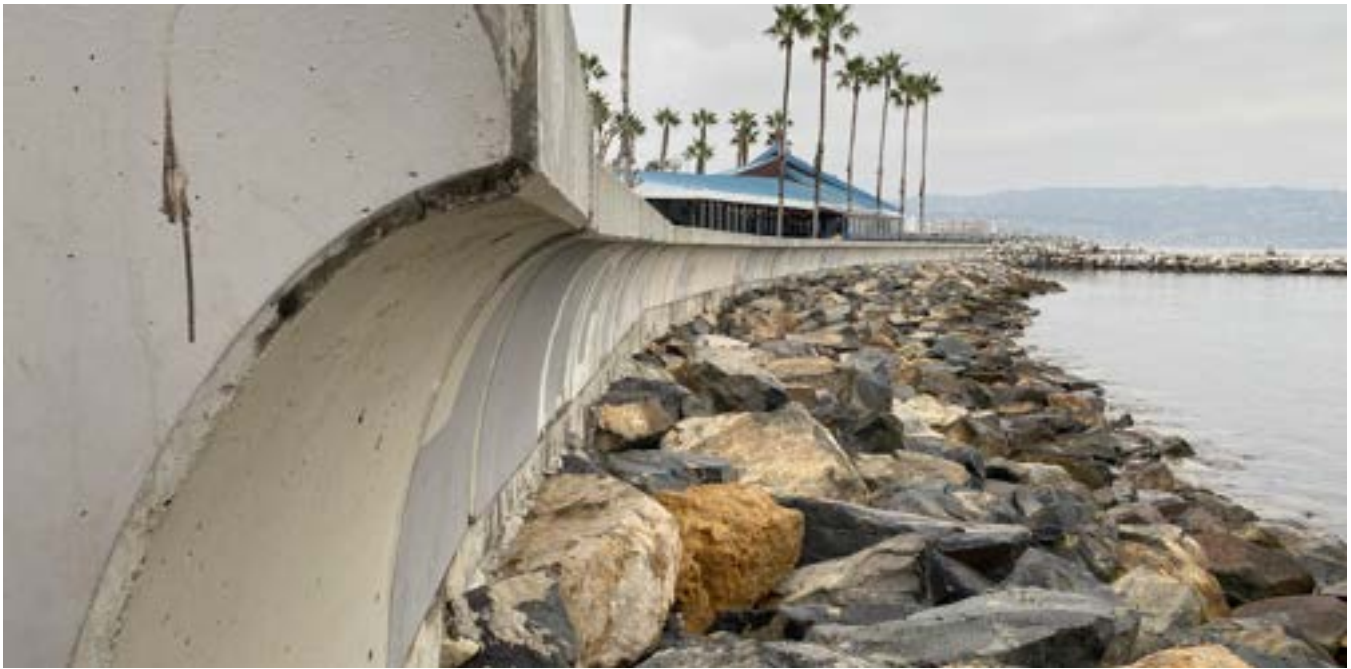
The splash wall that runs along the waterfront path through Mole D
