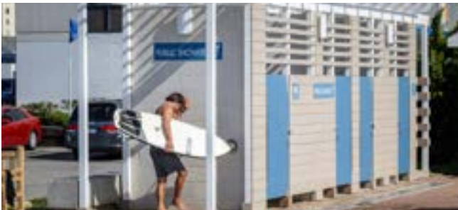
Bathroom facade with natural tones
