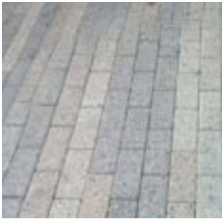
Brick pavers in running bond
