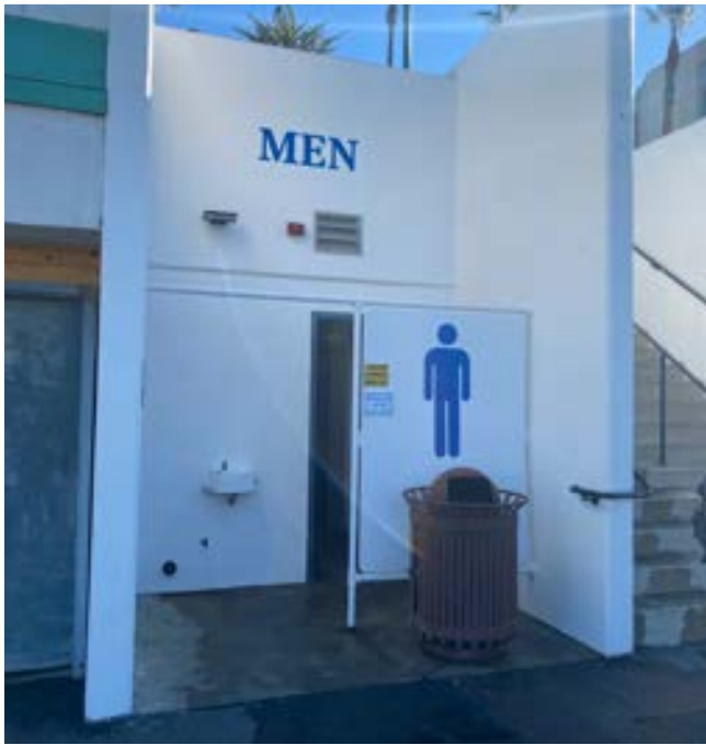
International Boardwalk Public Restrooms near stairs
