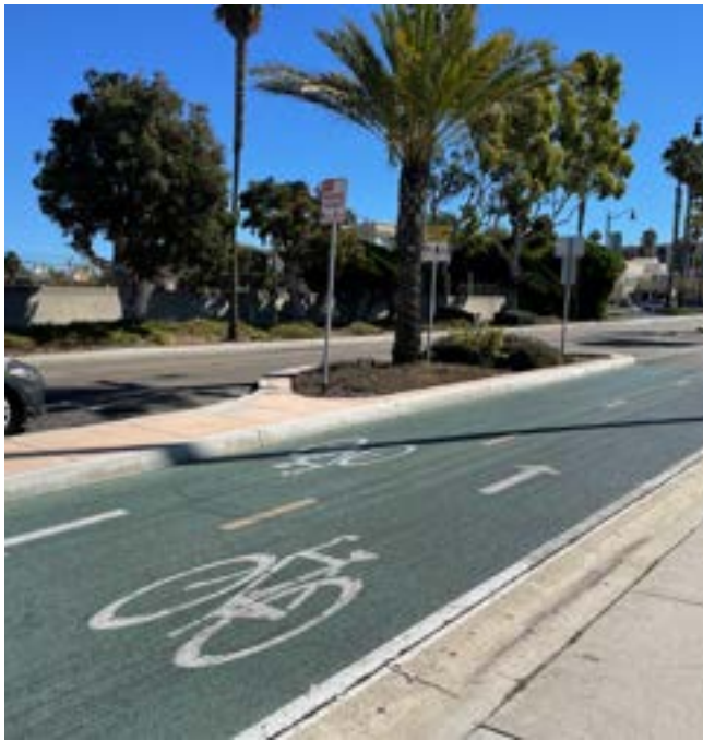
Two-way bike lane at North Harbor Drive
