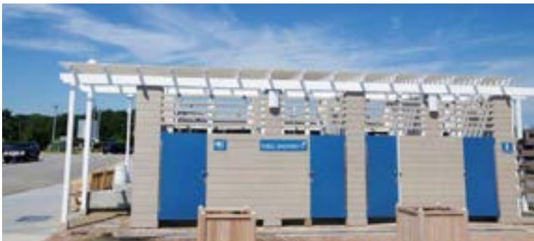
Bathroom facade with natural tones
