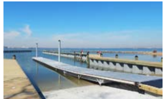
Concrete boat launch
