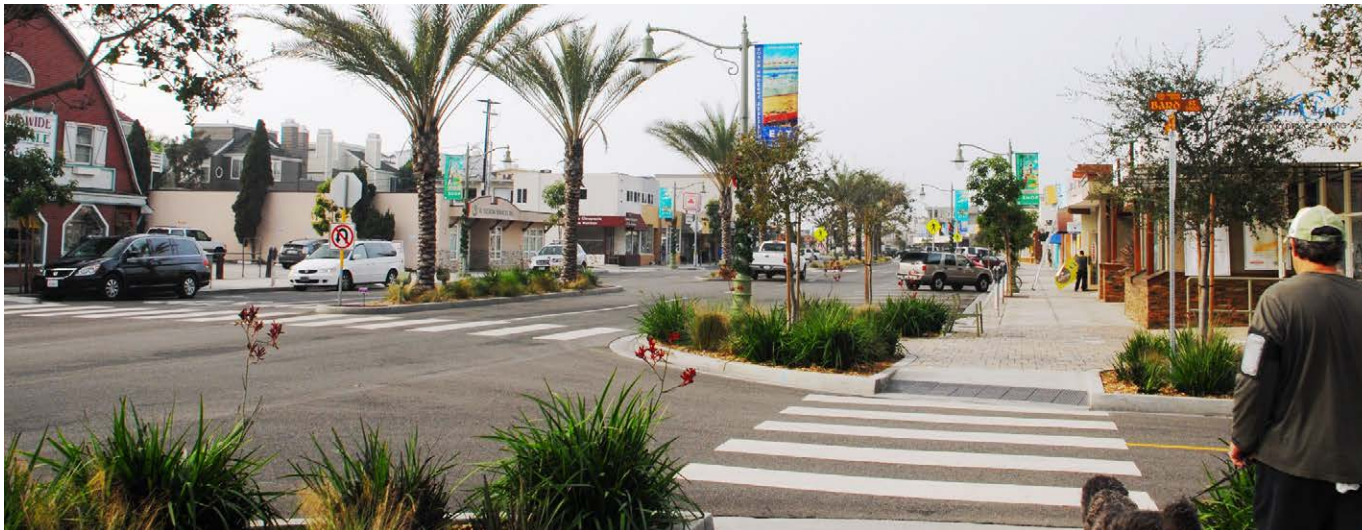
Bulb-outs at crosswalks with high-visibility continental striping improve pedestrian safety by limiting exposure to vehicles.
