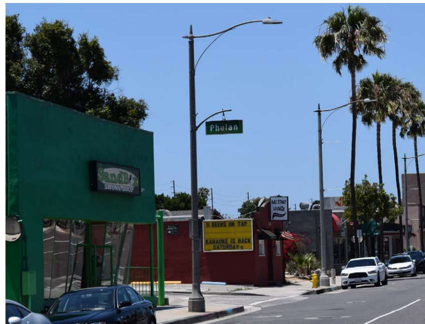
The mix of building types and setbacks and the inconsistent landscaping and signage design contribute to the Artesia Corridor's disjointed appearance.
