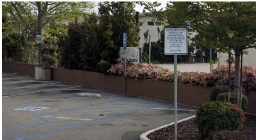
A pedestrian pass-through in this concrete block wall separating parking areas along the Artesia Corridor would improve pedestrian connectivity.
