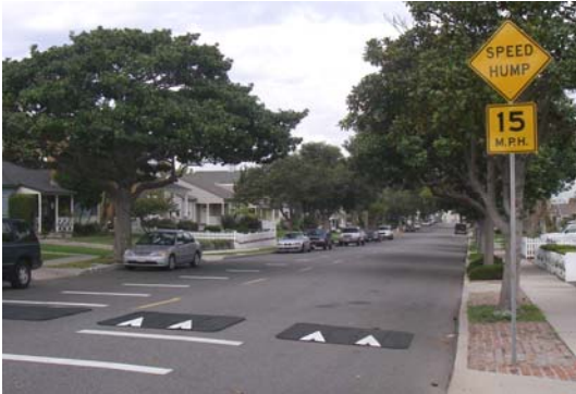
Speed cushions have been installed on Avenue E in Redondo Beach.
