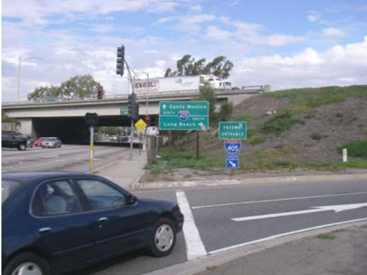
I-405 ramps at Inglewood Avenue
