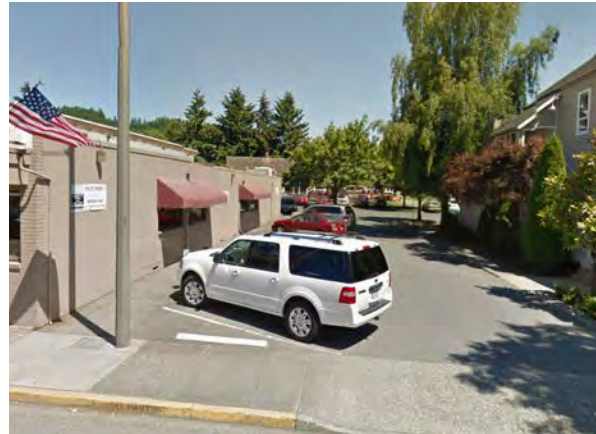
Parking to the side and rear of a building rather than the front allows for a more complete street frontage and an identifiable retail experience.
