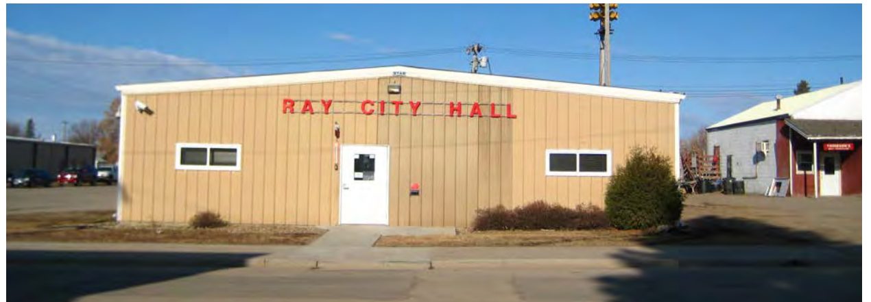
Existing City Hall
