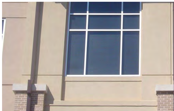
Pilasters (column projecting from a wall) and reveals (feature that creates an inset edge) create interesting shadows and add variety to a facade.
