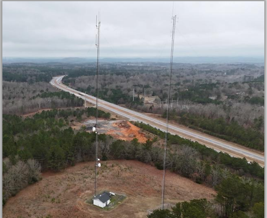
Figure 5. Radio Tower Site in Cedartown.
