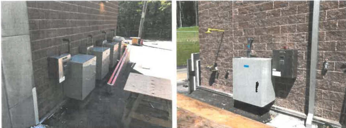
Figure 1 Chemical Fill Stations Complete
