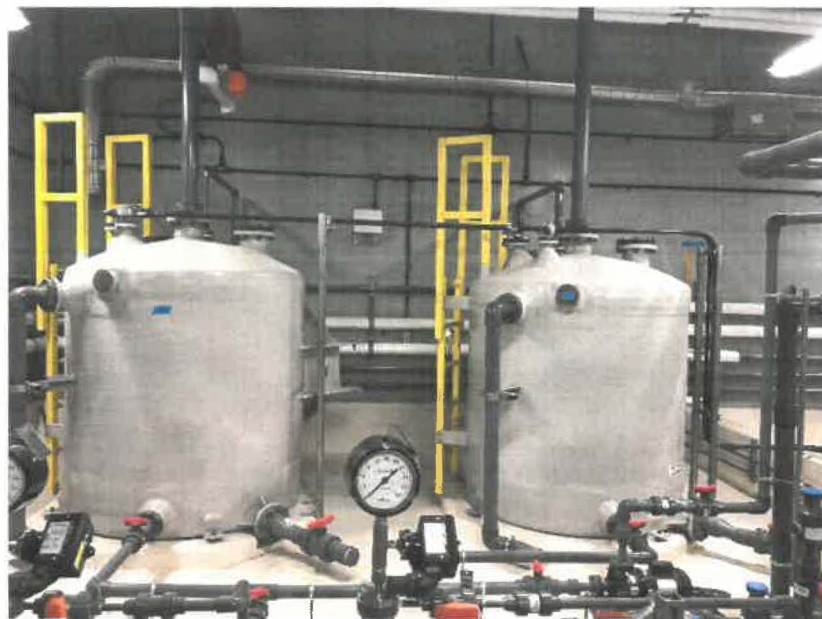
Figure 4 Sodium Hypochlorite Storage Tanks
