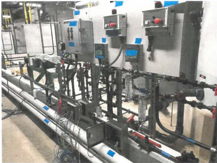
Figure 5 Chemical Metering station Wiring in Progress
