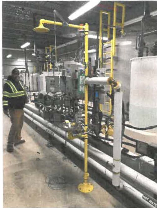
Figure 3 Emergency Eye Wash Station
