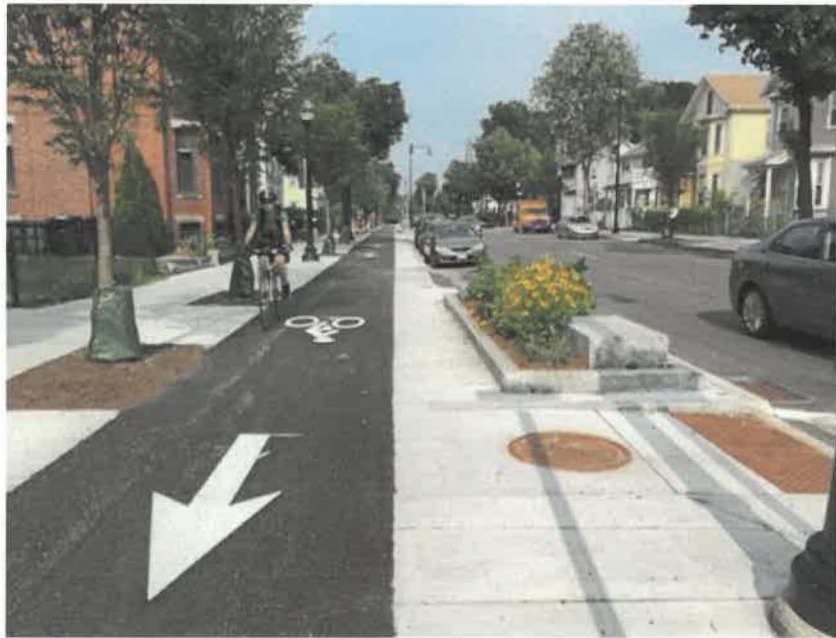
Western Avenue, Cambridge, MA Image Source: City of Cambridge, MA
