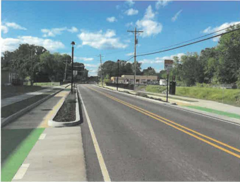
El Paso Avenue, Russellville, Arkansas Image Source: FHWA
