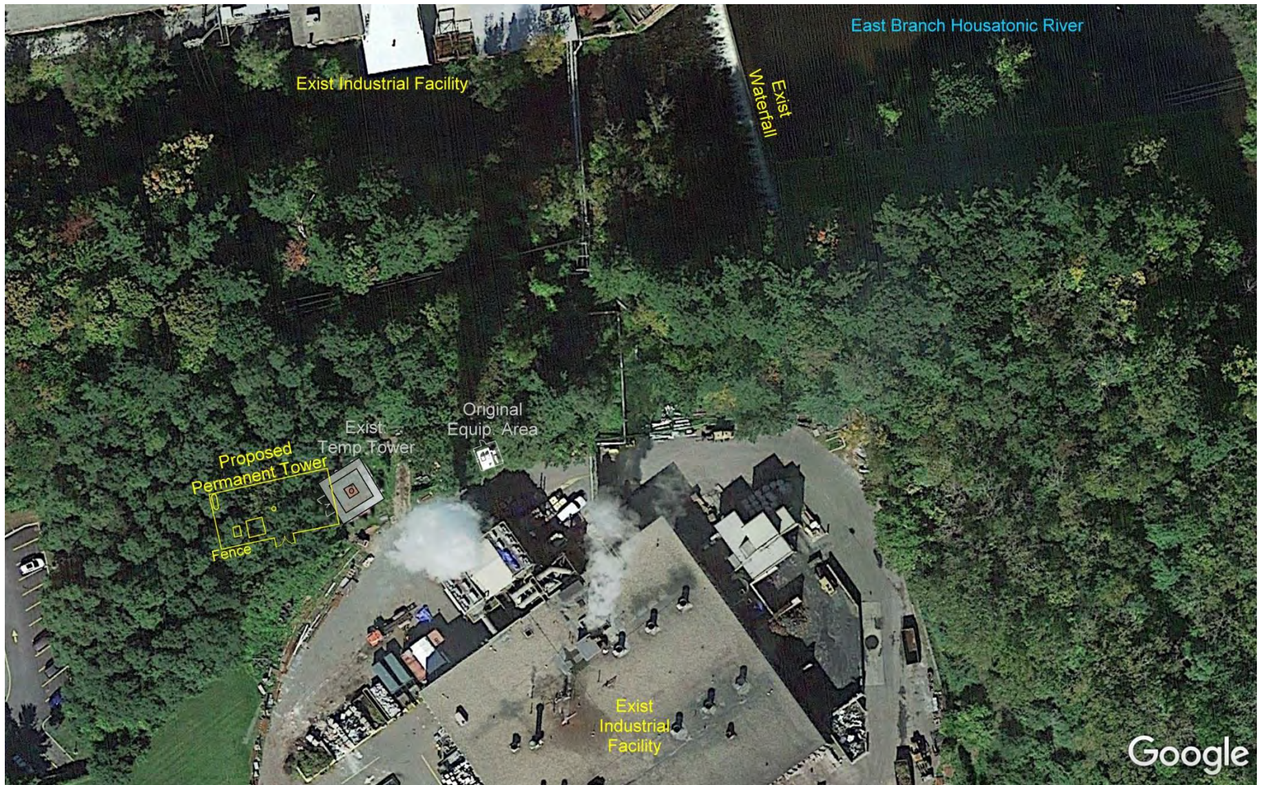
Figure 1: Aerial View of the Existing Industrial Facility Showing the Existing and Proposed Tower Locations.
