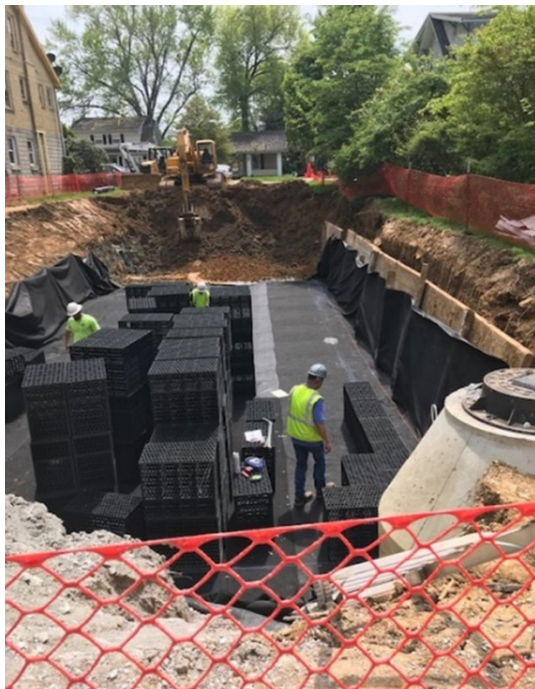
Figure 39: 20 th Street Stormwater Retention Project
