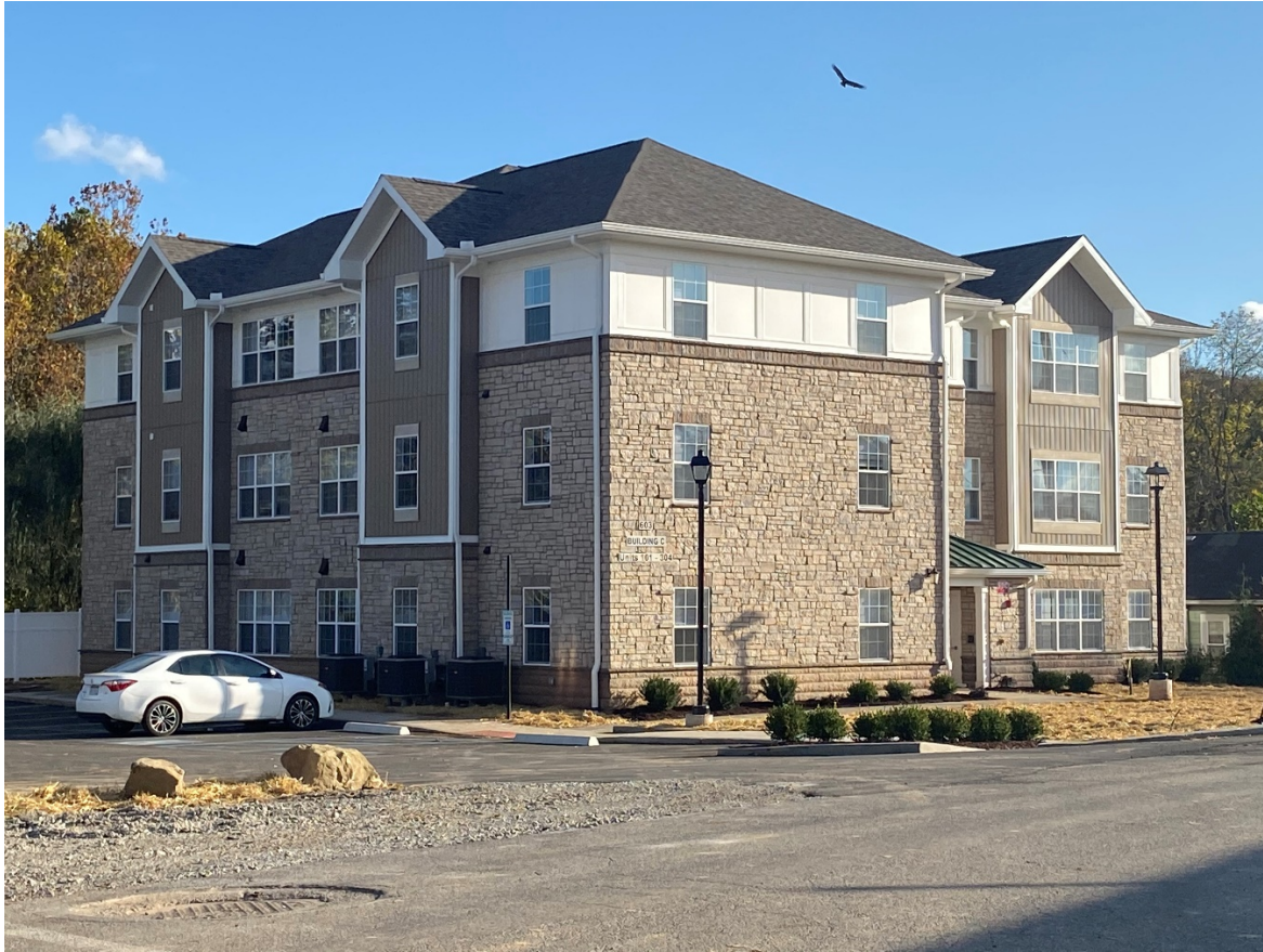
Figure 44: Rowan Apartment Complex on Buckeye Street
