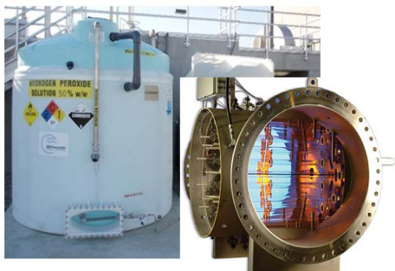
Example hydrogen peroxide feed tank and UV reactor
