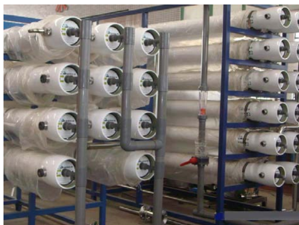
Example reverse osmosis membrane rack
