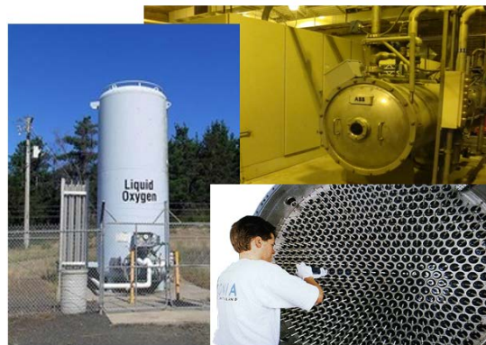
Example liquid oxygen tank and ozone generator system
