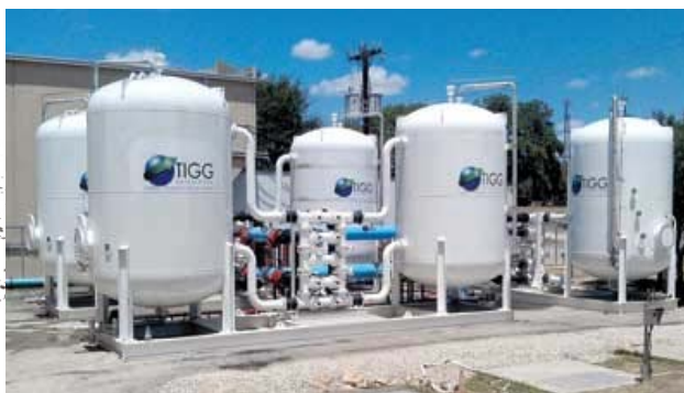
Example granular activated carbon pressure vessels
