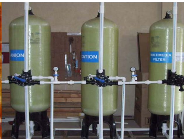
Example photo of ion exchange contactors
