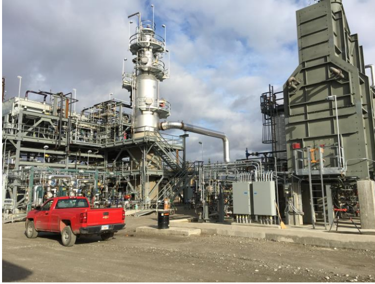
View of the Vacuum Heater (right) and Vacuum Tower installed as part of the Petro Star Asphalt Plant Project.
