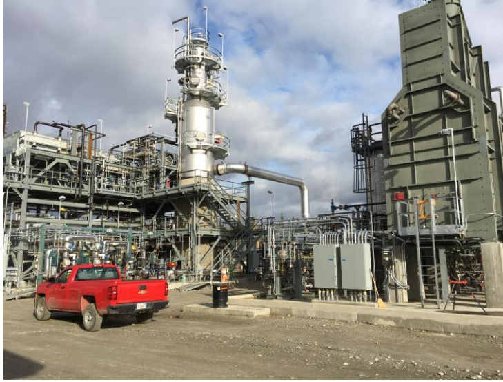
View of the Vacuum Heater (right) and Vacuum Tower installed as part of the Petro Star Asphalt Plant Project.
