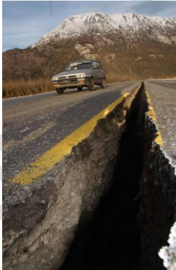
Figure 8-1: Denali Earthquake Road Damage
